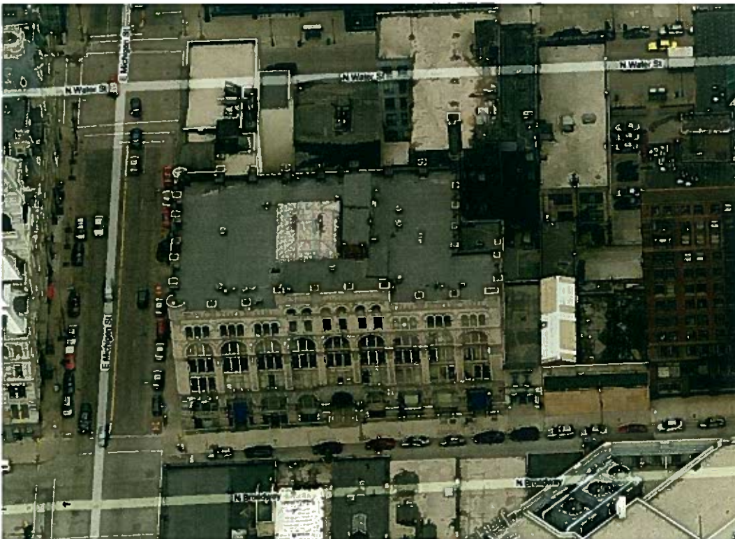
Photo 2: Aerial Looking West
