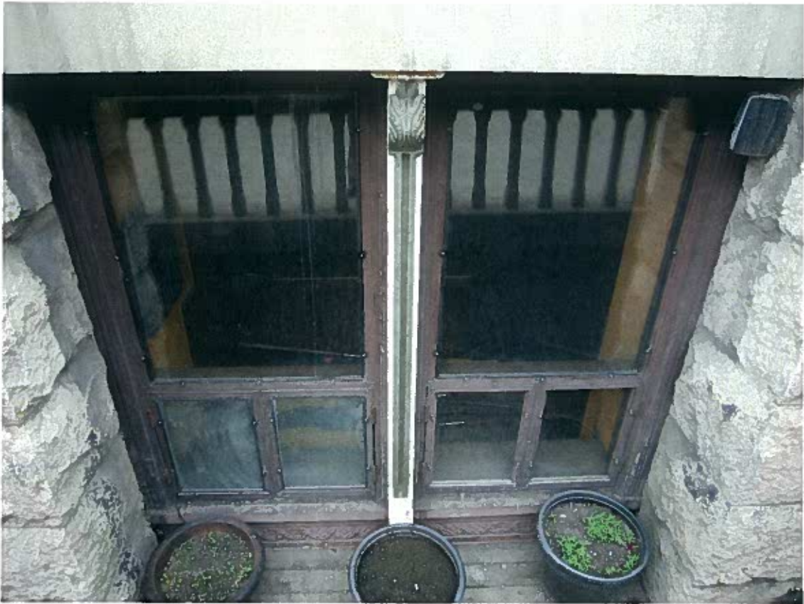
Photo 17: Ground Floor window detail
