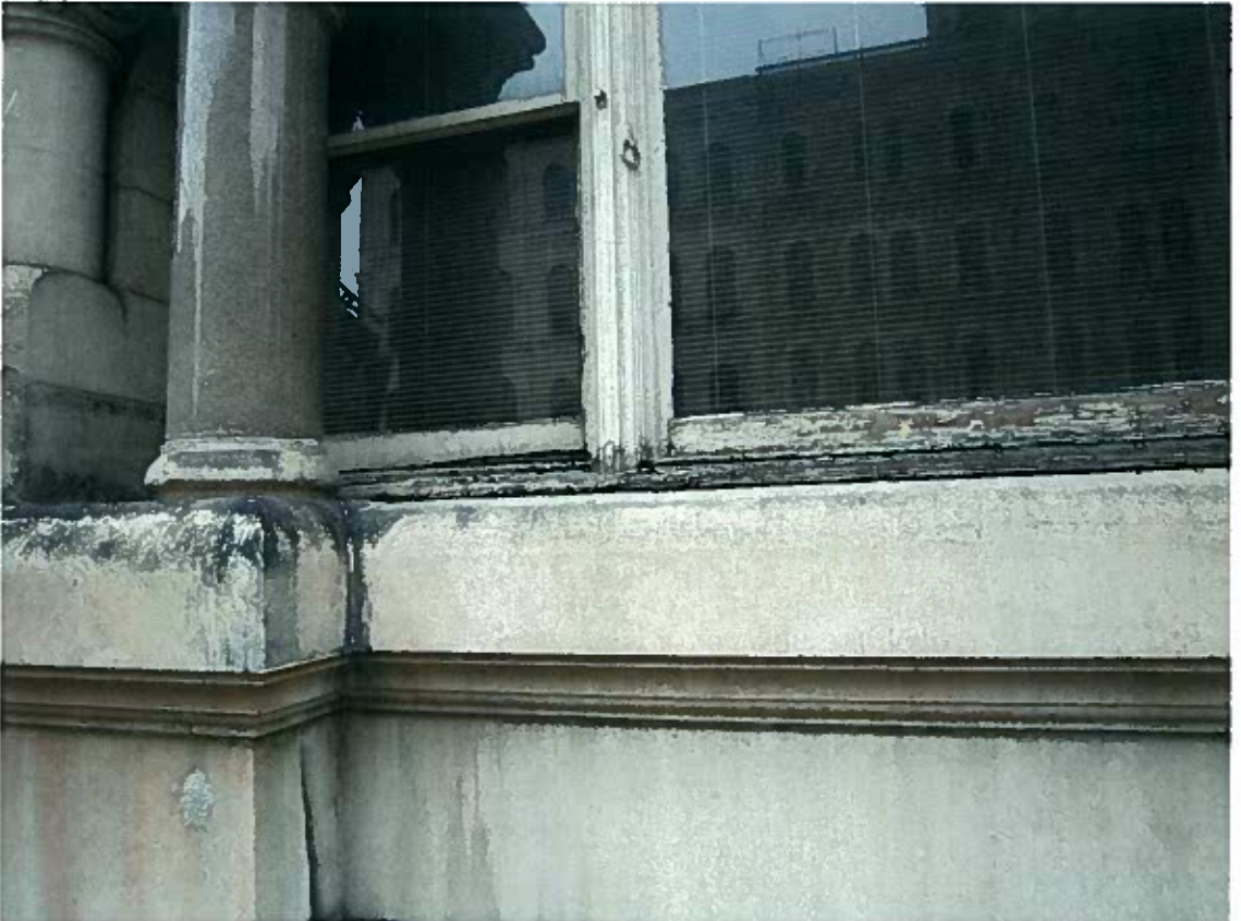
Photo 20: Typical window condition
