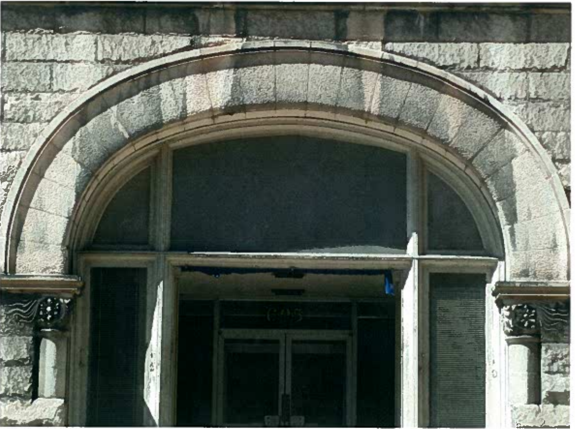
Photo 16: First Floor window detail
