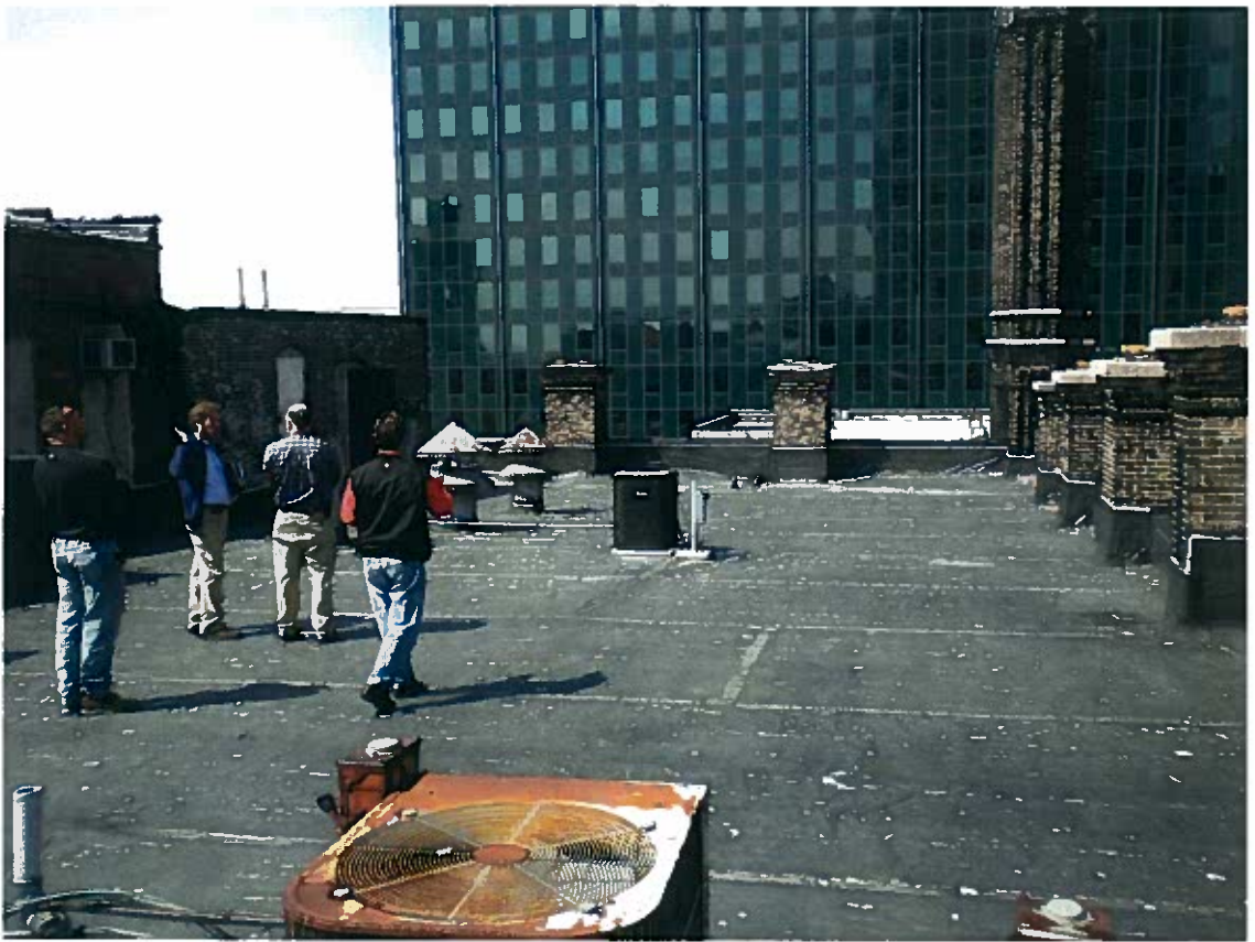
Photo 19: Roof, looking West
