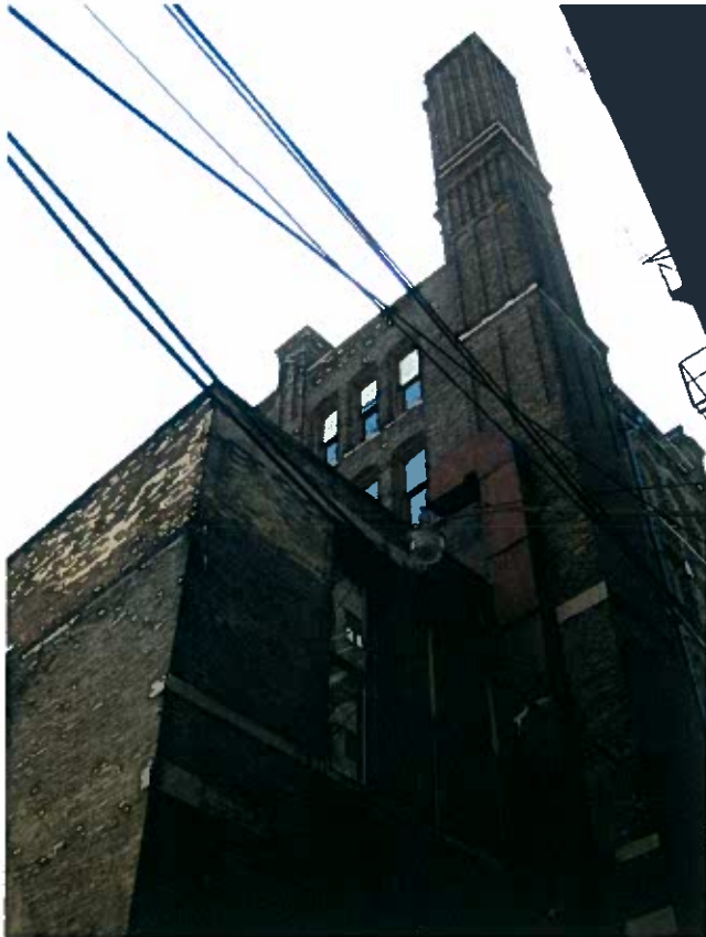
Photo 10: Alley Façade, looking South
