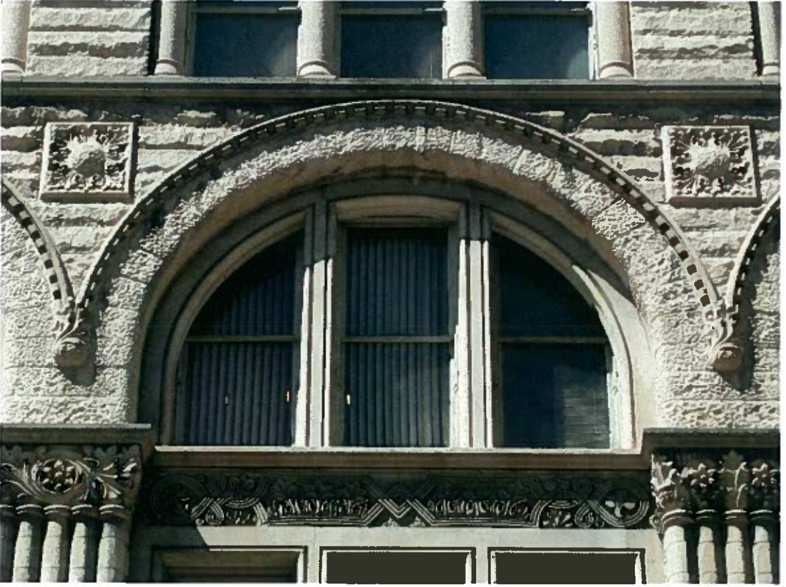
Photo 14: Fourth Floor window detail
