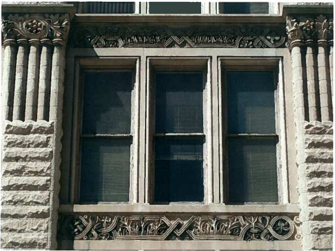
Photo 15: Third Floor window detail
