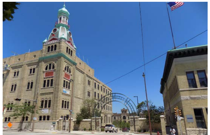
Office Buildings in Schlitz Park
