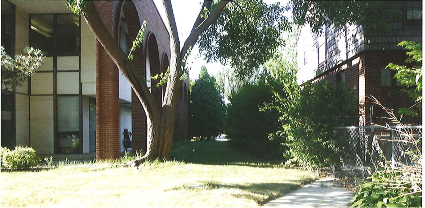
VIEW LOOKING NORTH ALONG EAST PROPERTY BOUNDARY AT WEST STATE STREET
