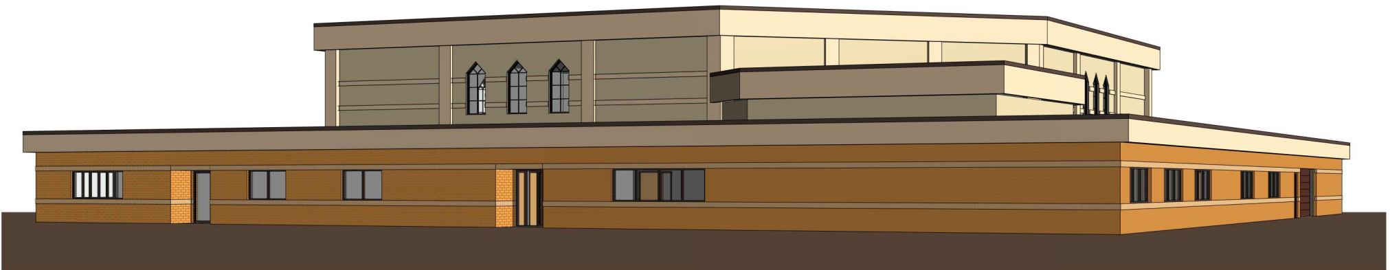
View from N. 73rd St
