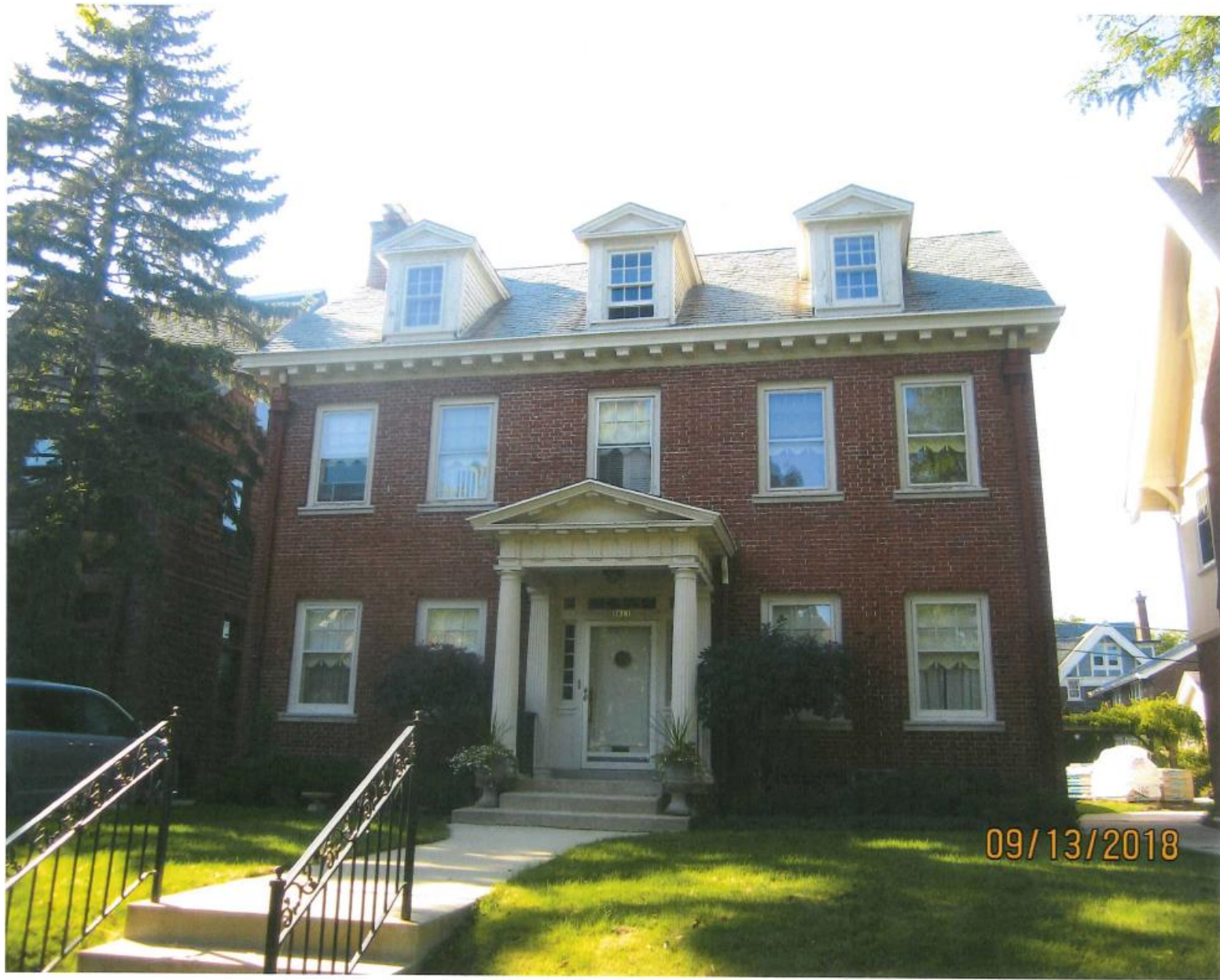
Work area is the three front dormers.
