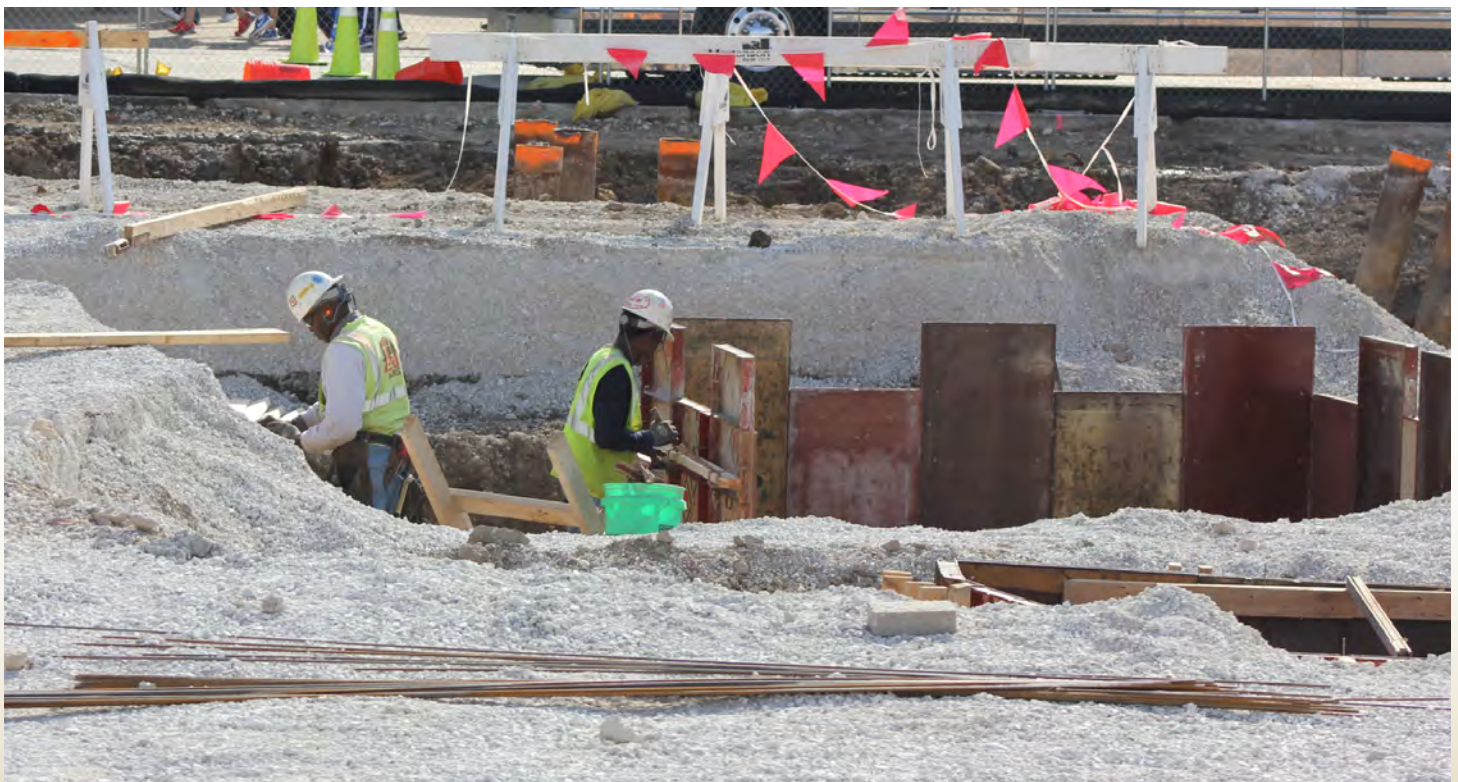
Workers setting forms for concrete pour.
