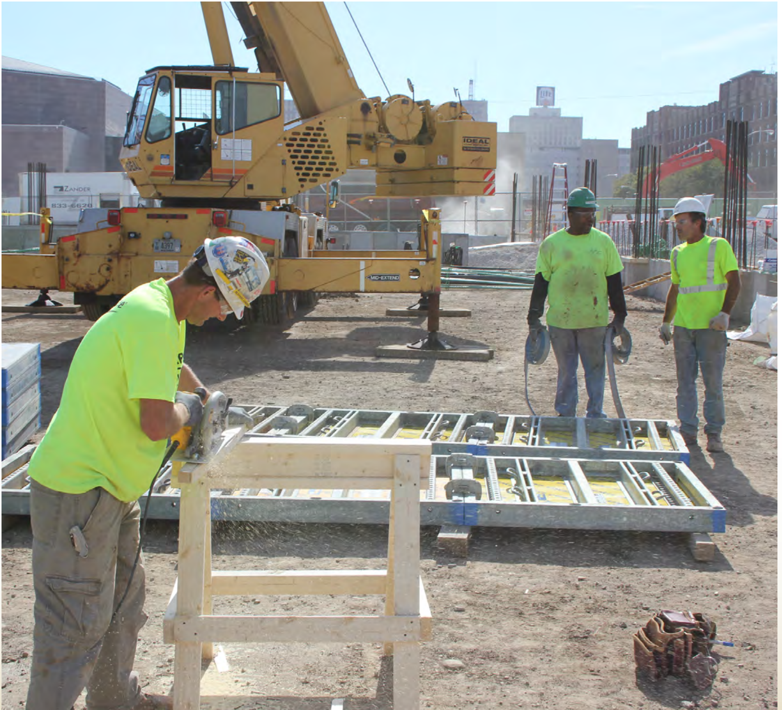
Laborers working on the Block 7 Parking Structure site.
