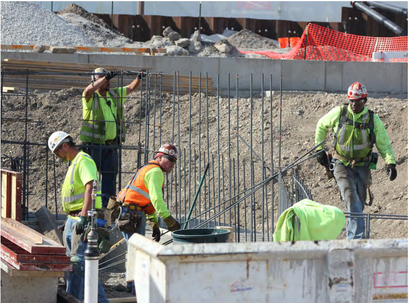
Ironworkers preparing rebar for concrete pour on the New Milwaukee Arena
