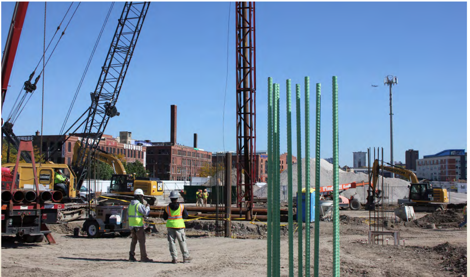
Workers monitoring the pile driver.
