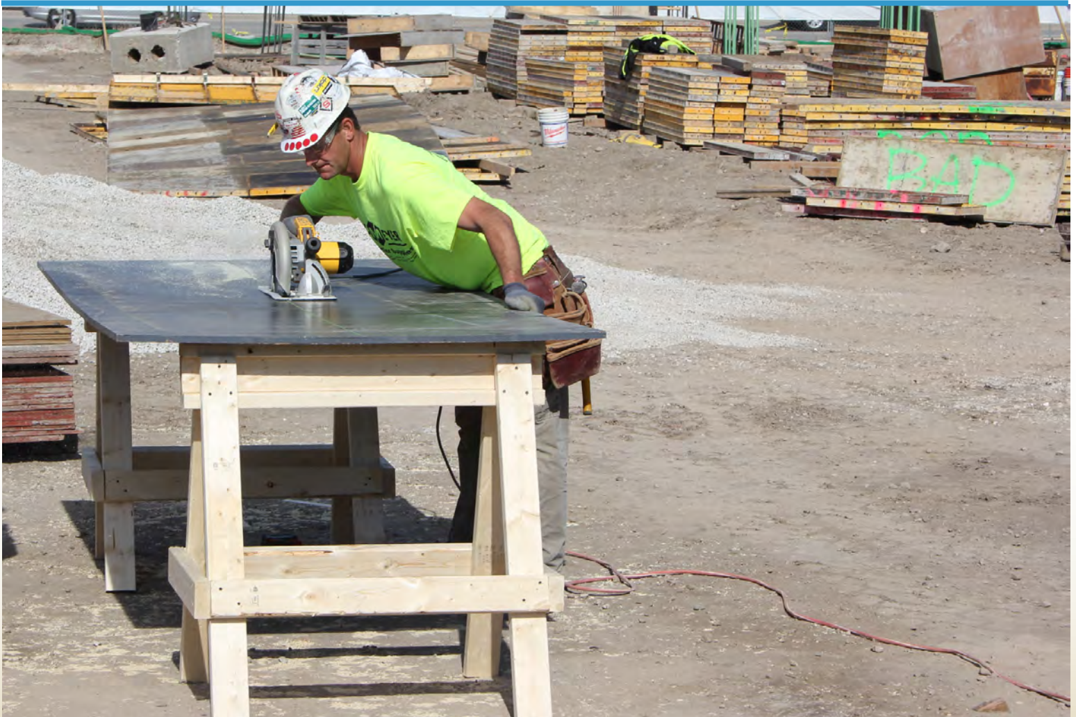
Journeyman Carpenter cutting concrete form to size.
