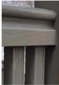
Existing Handrail (Front Porch)
