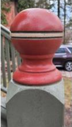
Existing Post Finial (Front Porch)
