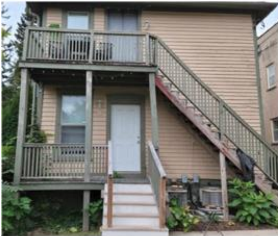
Existing Rear Elevation (Prior to stair failure and demo)
