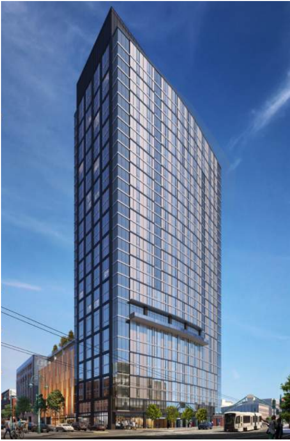
333 N. Water Street Milwaukee (under construction)
