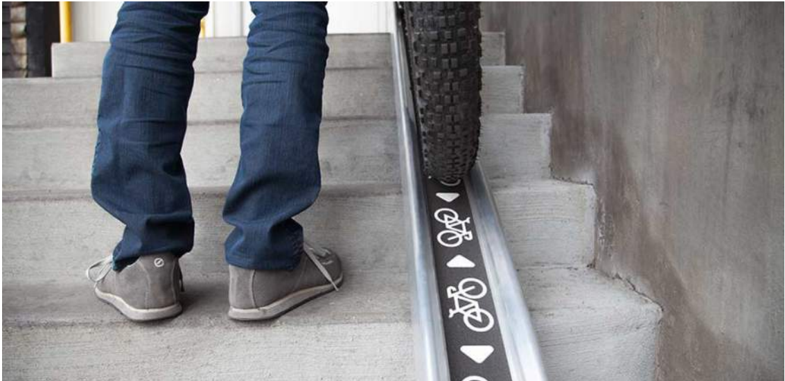
Bicycle Access Ramp Example
