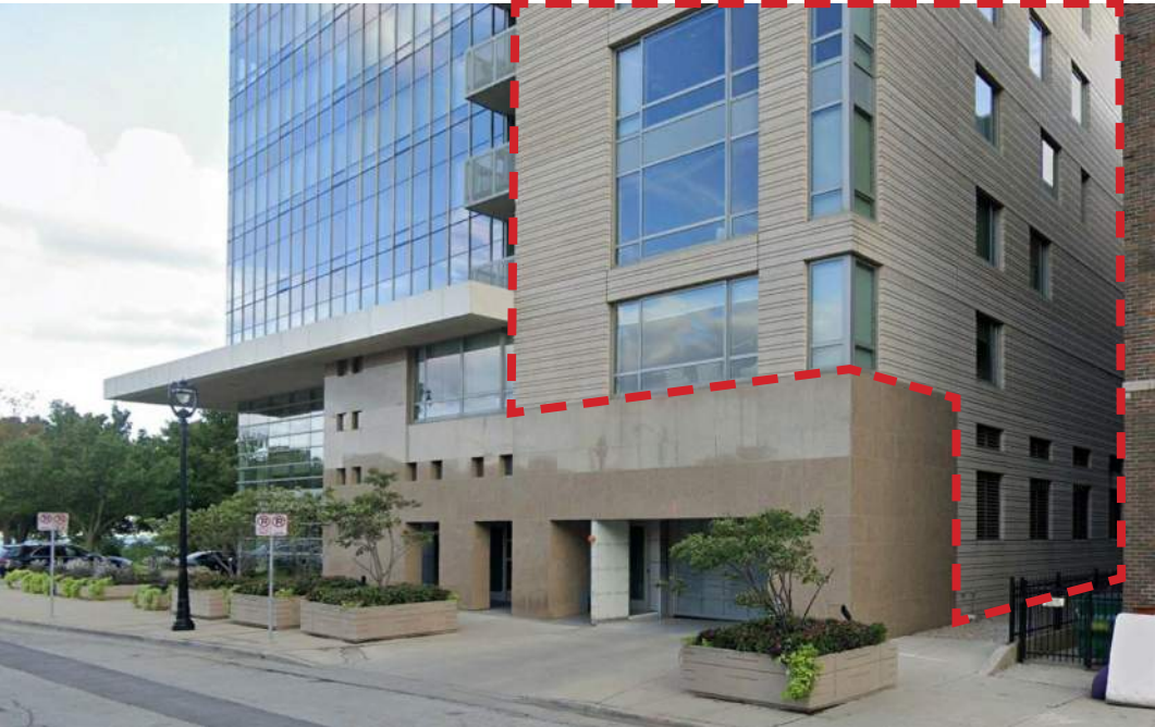
Precast Panel used in Kilbourn Tower
