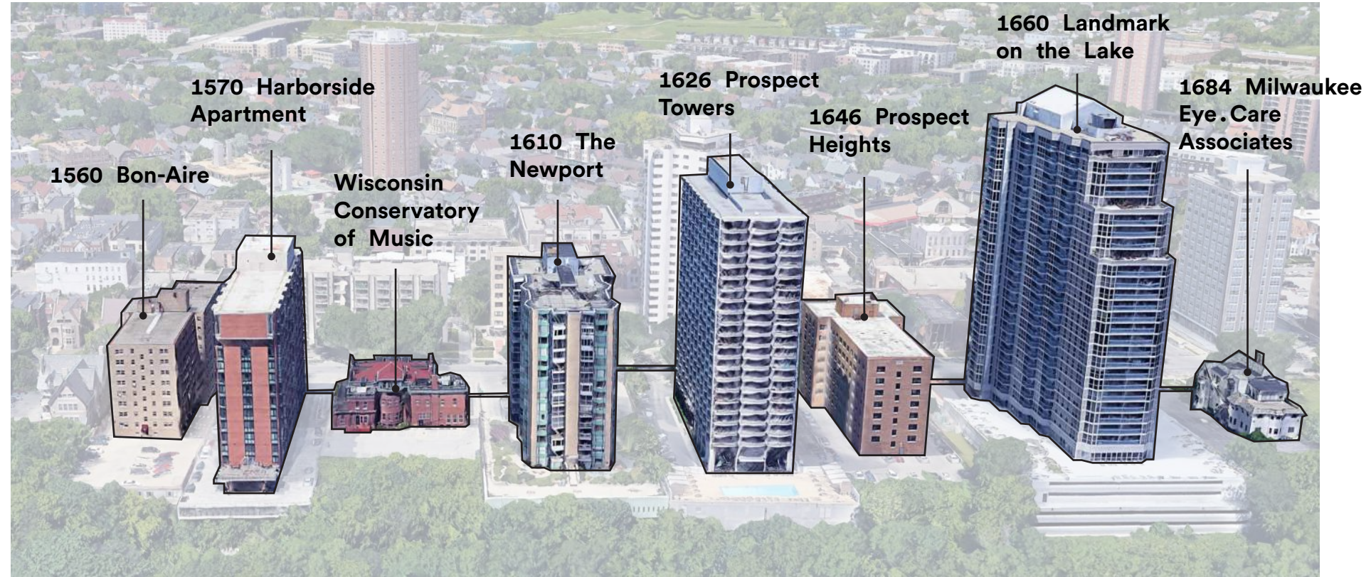
Tower Separation Distance along N. Prospect Avenue (#1684 - #1560)
