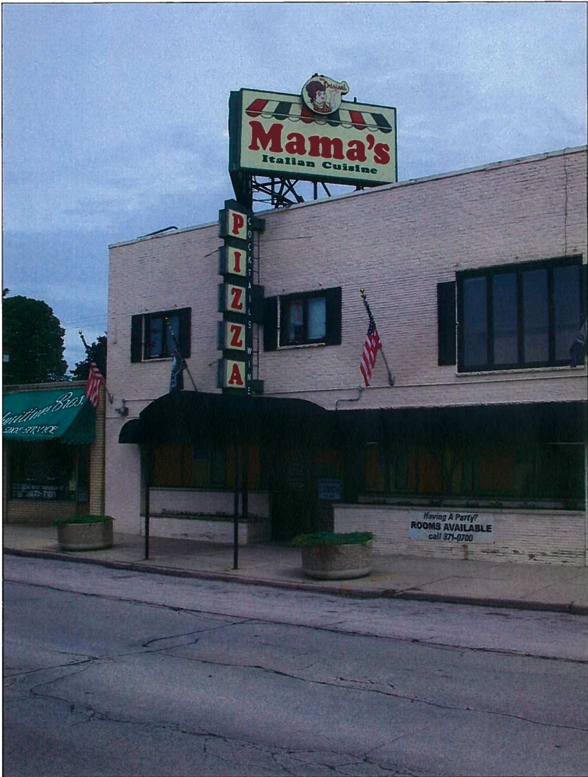
CCF 091114 7718-20 W Burleigh St 6-2-2010 Looking NW'ly from median in Burleigh at west covered walk a two of the moveable planters.
