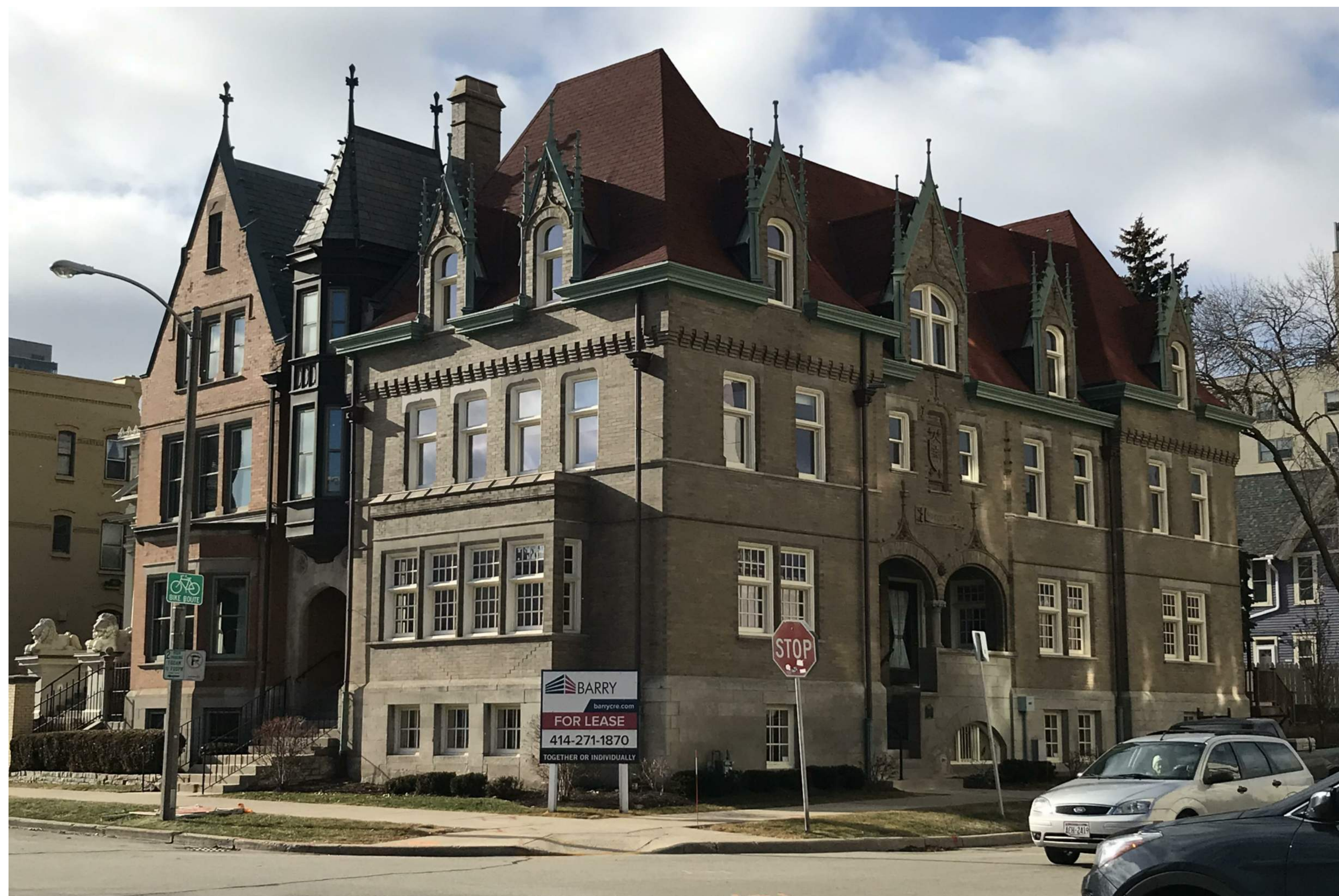
HISTORIC PHOTOGRAPH - EXISTING CONDITIONS 1 1/2" = 1'-0"
