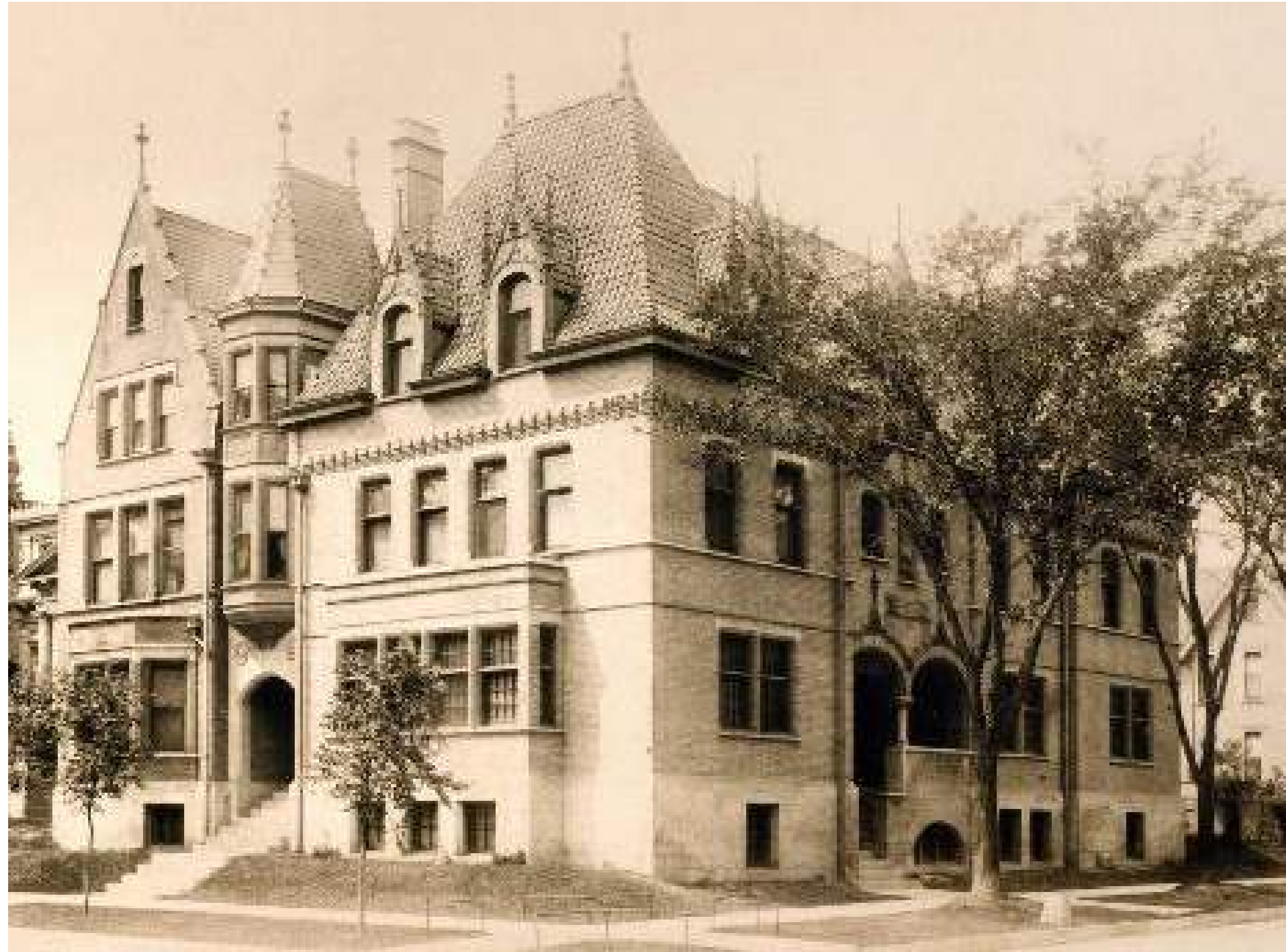
BLOODGOOD HOUSE WITH CLAY TILE ROOF. 3 HISTORIC PHOTOGRAPH - CLAY TILE 1/2" = 1'-0"
