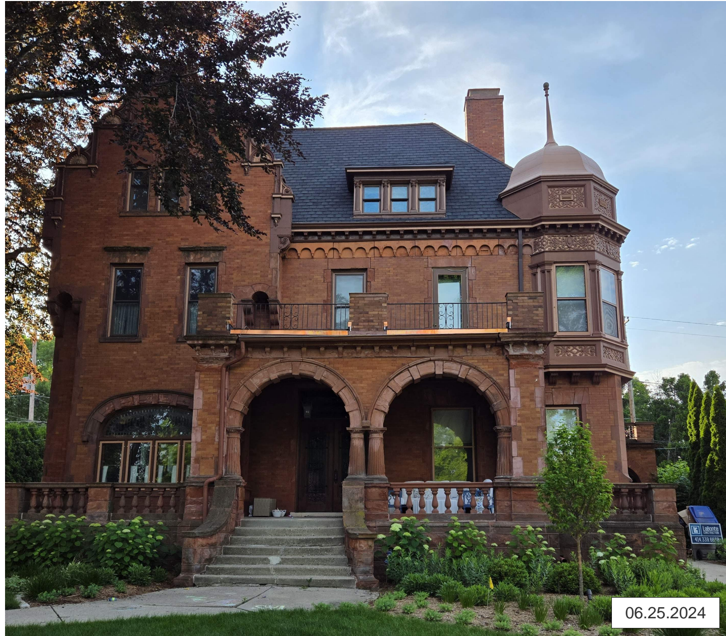
CURRENT ASPHALT SHINGLE ROOF
