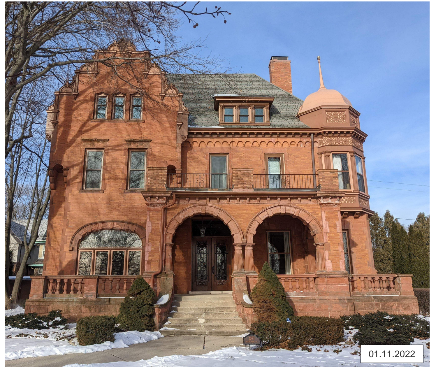
PREVIOUS ASPHALT SHINGLE ROOF
