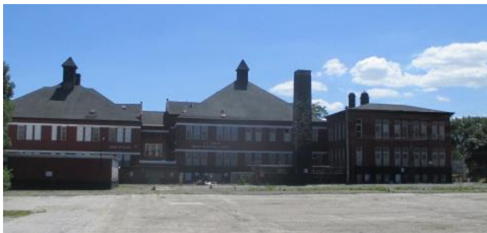
2001 West Vliet Street: North Elevation
