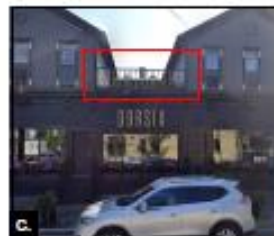
New Decorative Wood Railings: Wood railings, posts, rails, balusters, railing caps and finishes to match existing wood railing located above Dorcia sign on the North face of the building.
