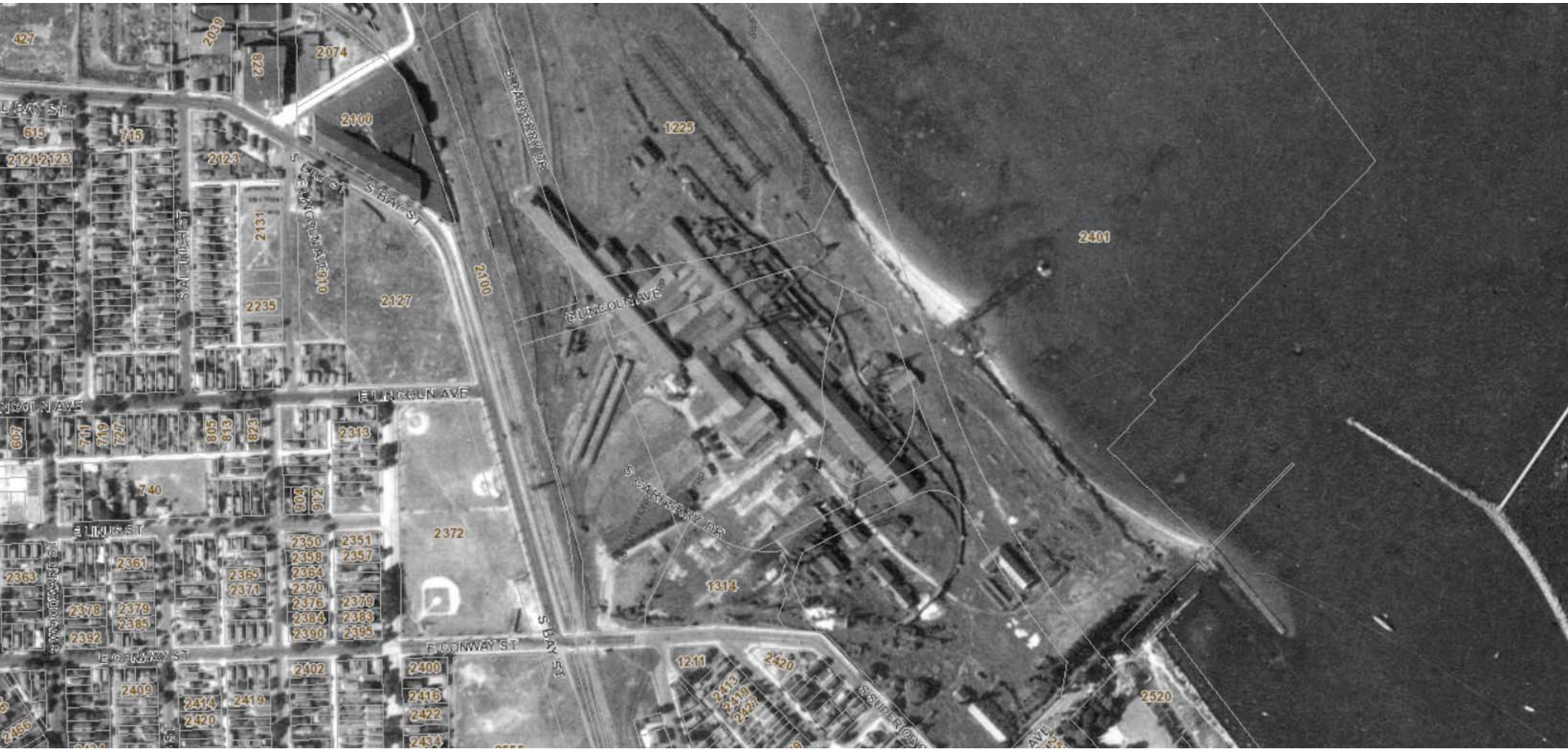
1937 AERIAL SHOWING THE STEEL ROLLING MILL
