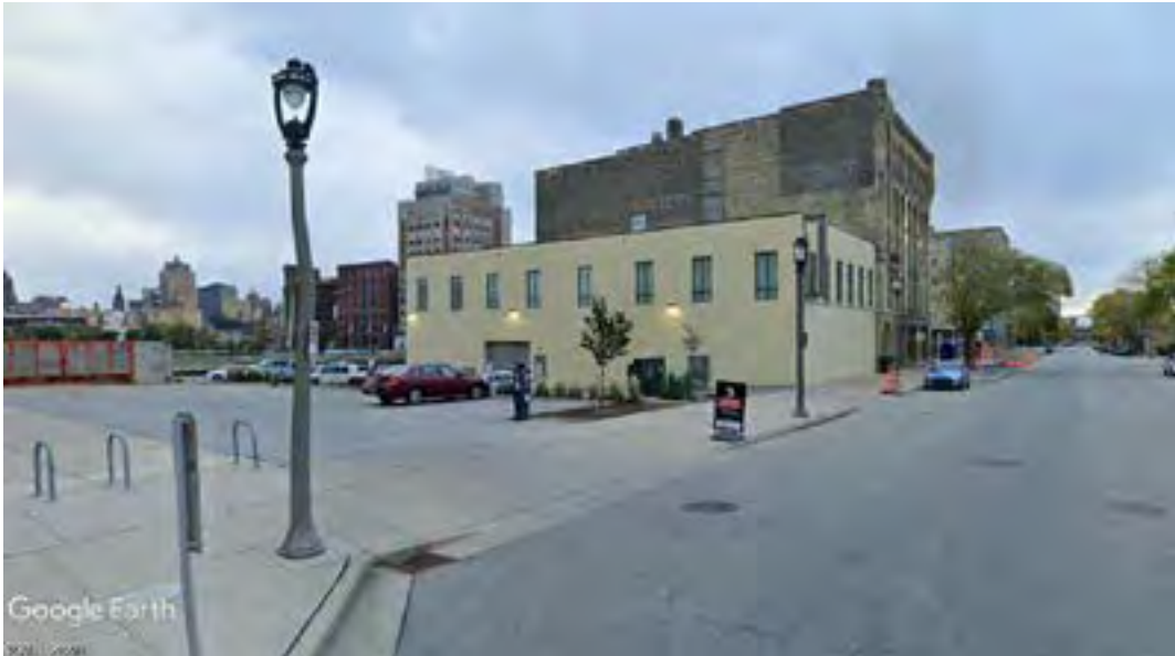
Looking NE from Florida Street and S. 4th Street (Source: Google Earth, 2019)
