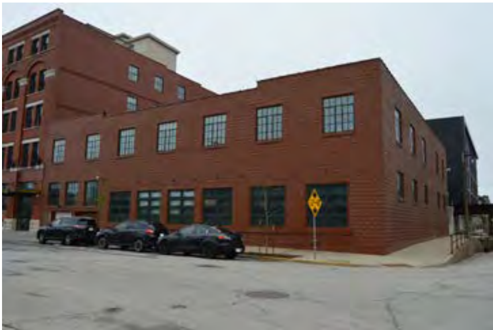
Two-story warehouse addition, looking southeast
