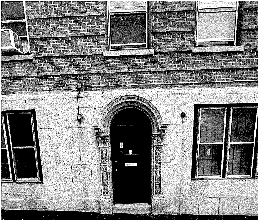
Service entrance on N. 31 st St.
