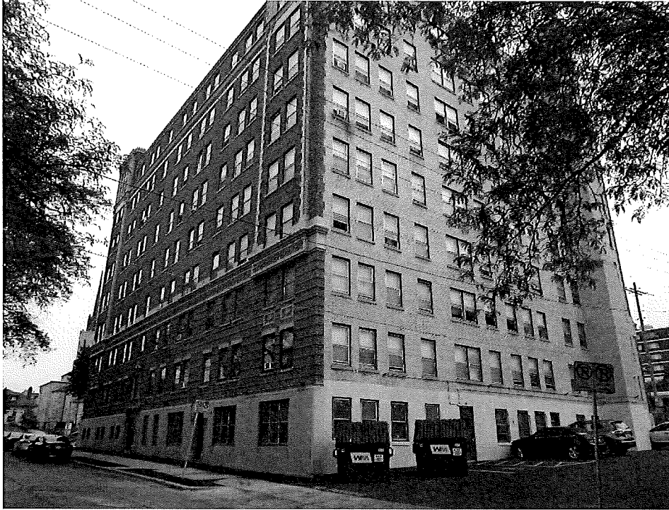
View looking northeast from N. 31 st St.
