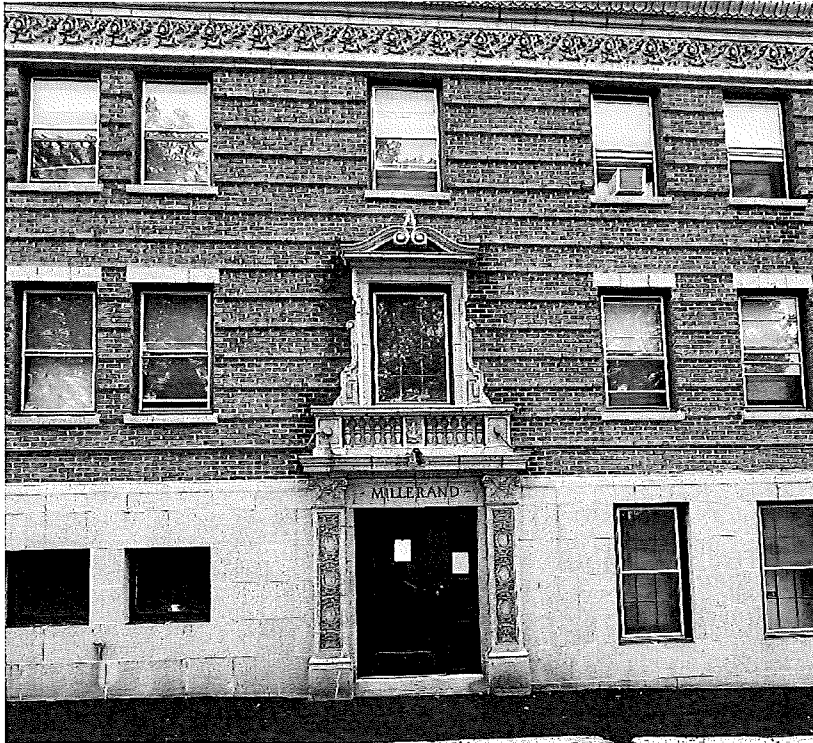
Details of west facade
