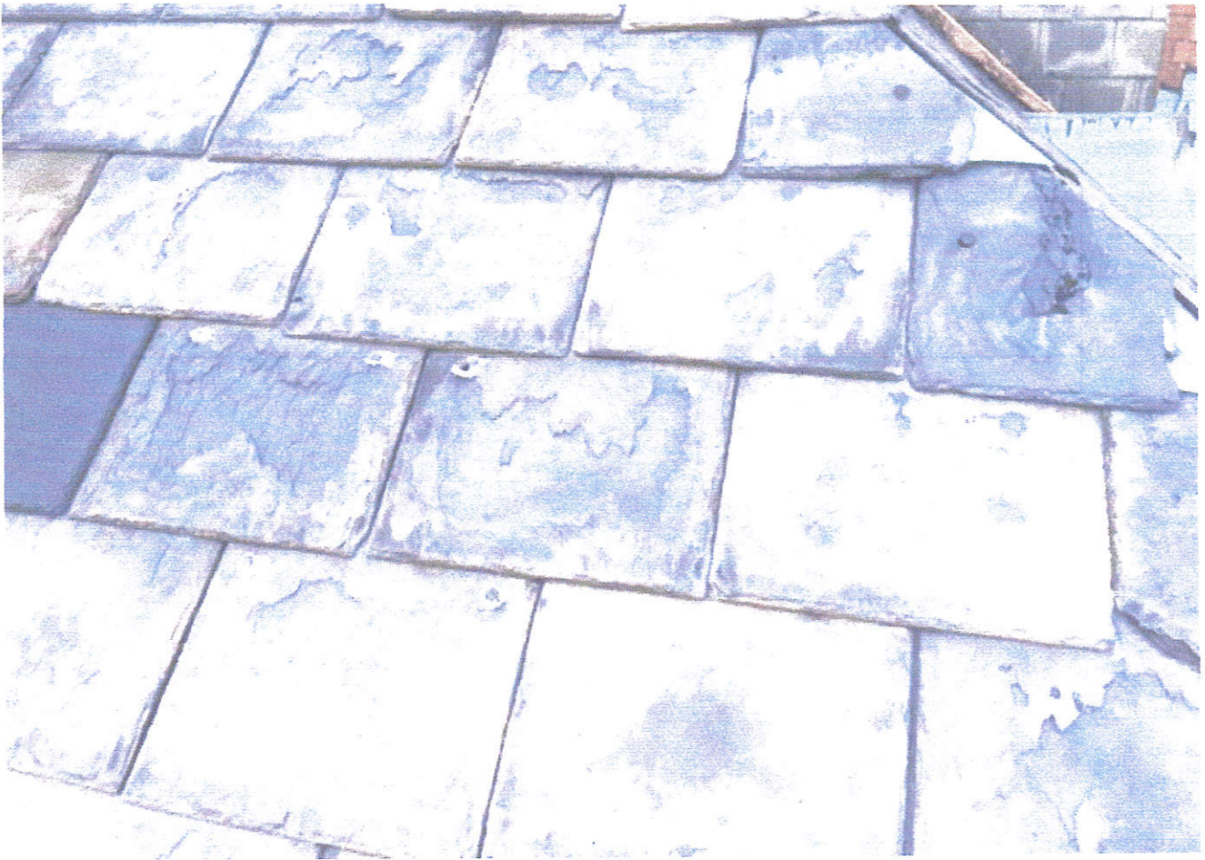
South Facing view of Roof at 3112 W. Kilbourn
