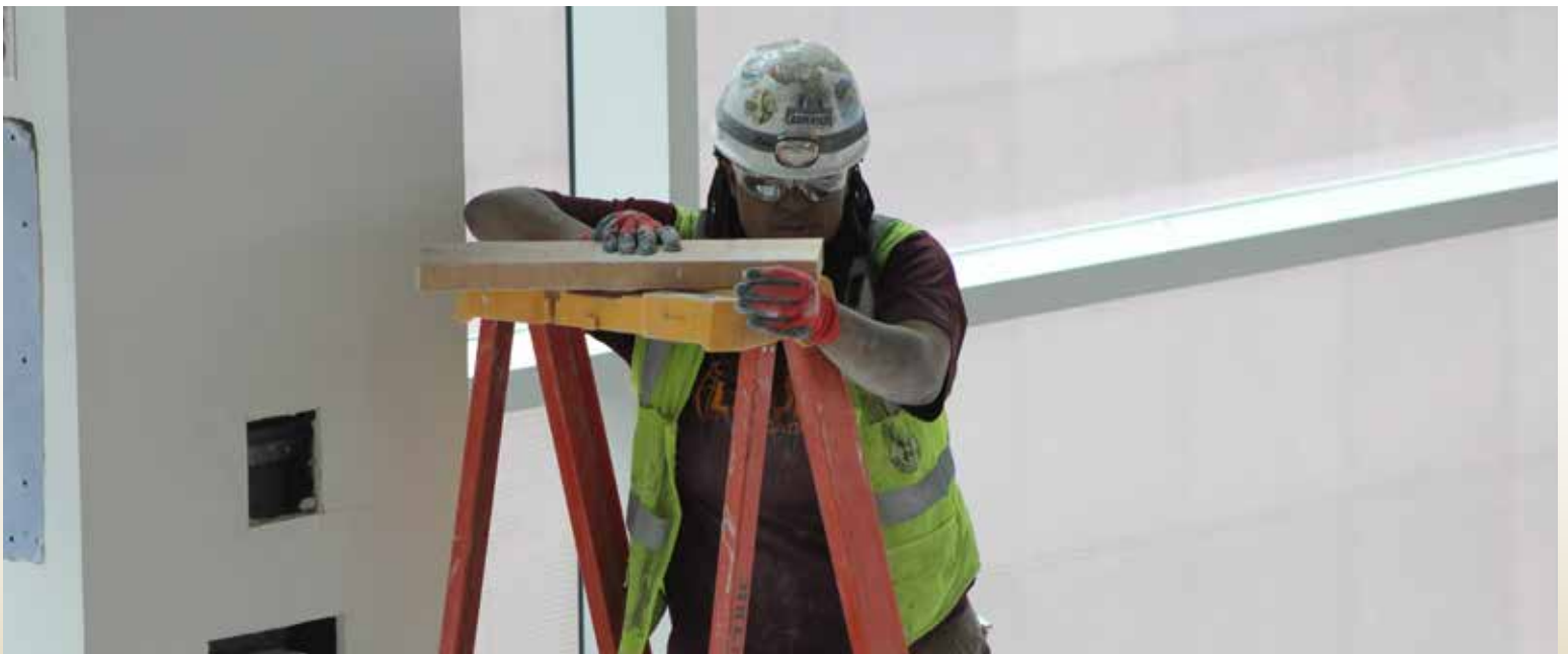
Worker installing electrical fixtures.
