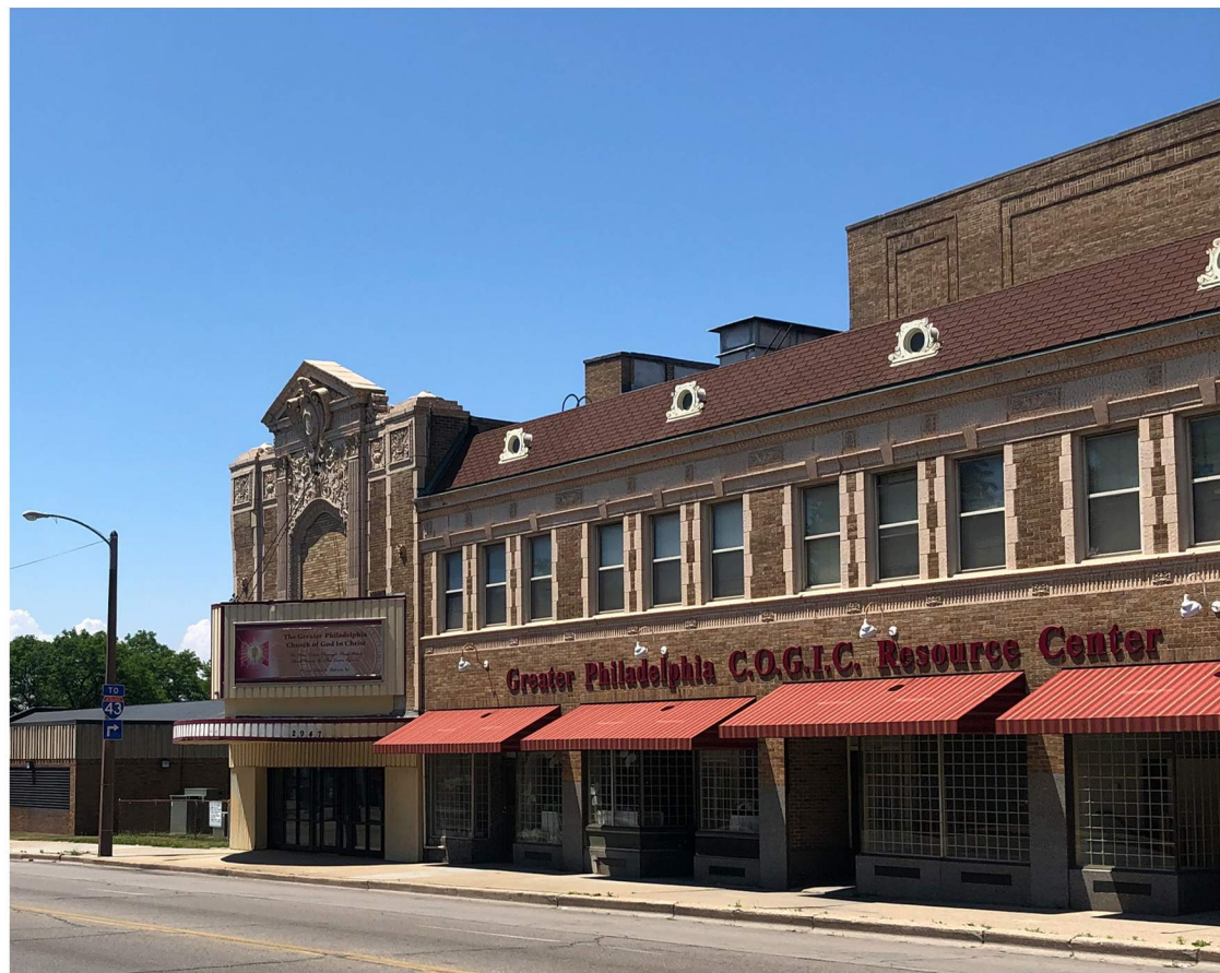
Storefront areas to be converted into walk up units
