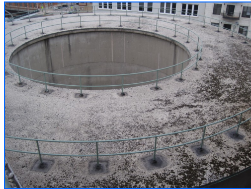
Roof at helical ramps
