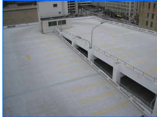
Light poles and fixtures at the eight floor
