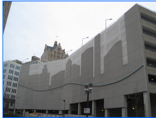
EIFS wall at north elevation
