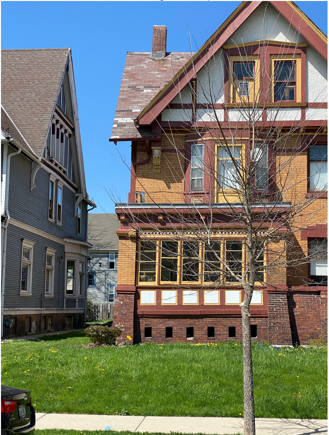
Side Profile of the House This is where the Air Conditioning Condenser is planned to be sited.
