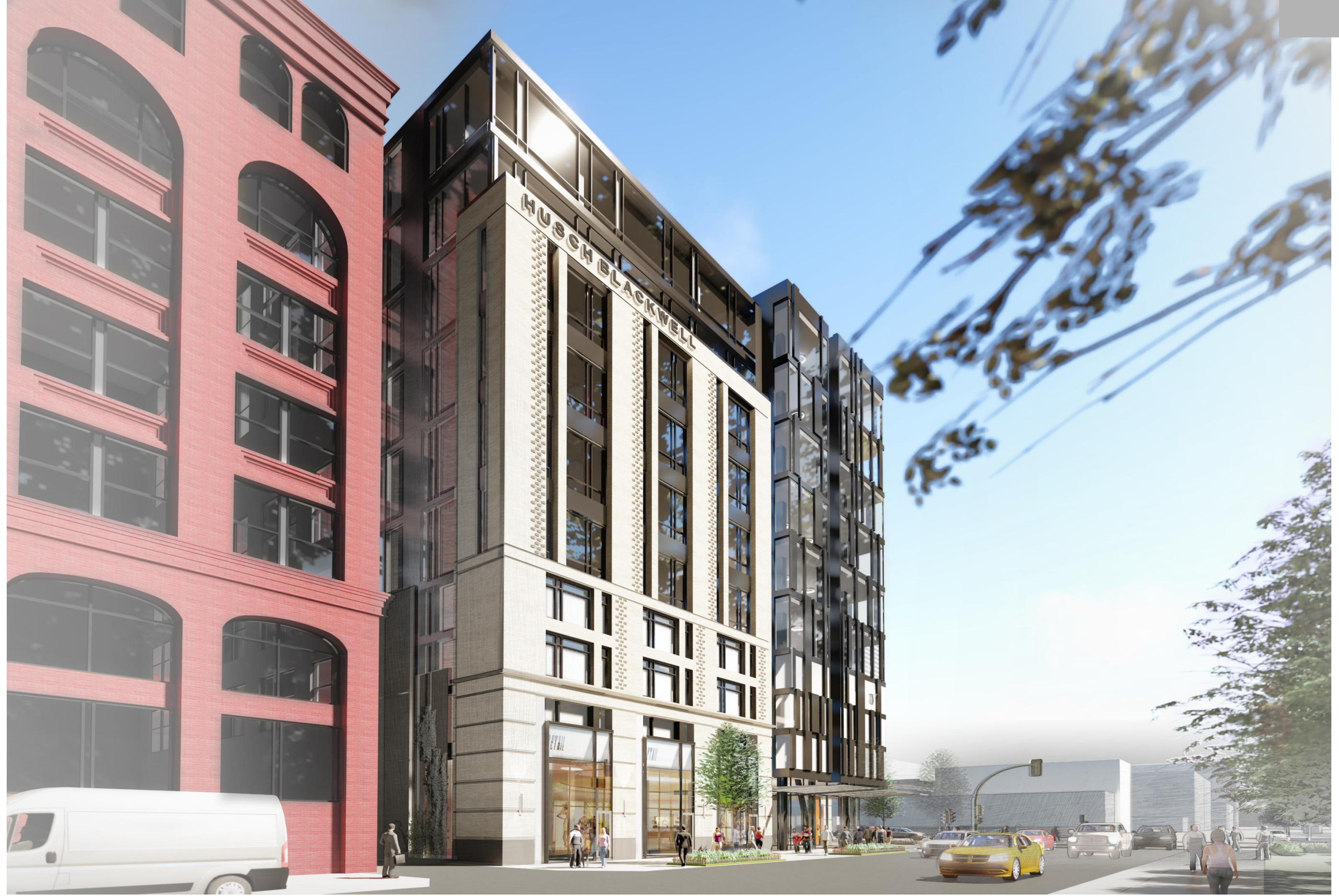
VIEW FROM SW
