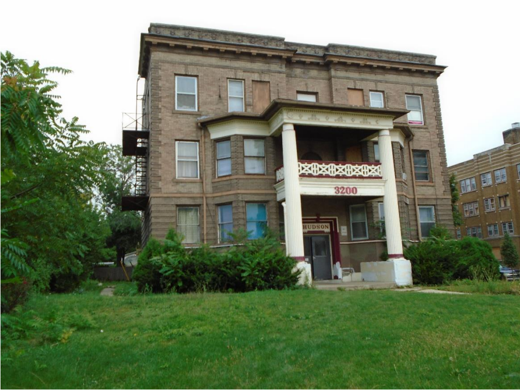
Hudson Flats Apartment Building. Photo taken 2015.
