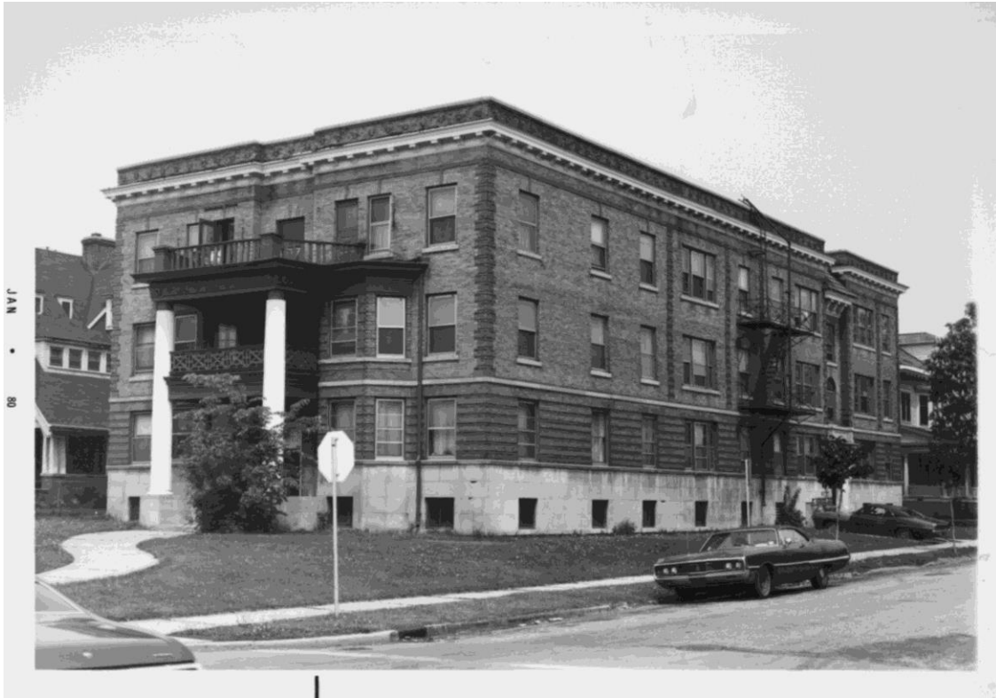
Wisconsin Architecture and History Inventory, Record #30295. Photo taken 1980.
