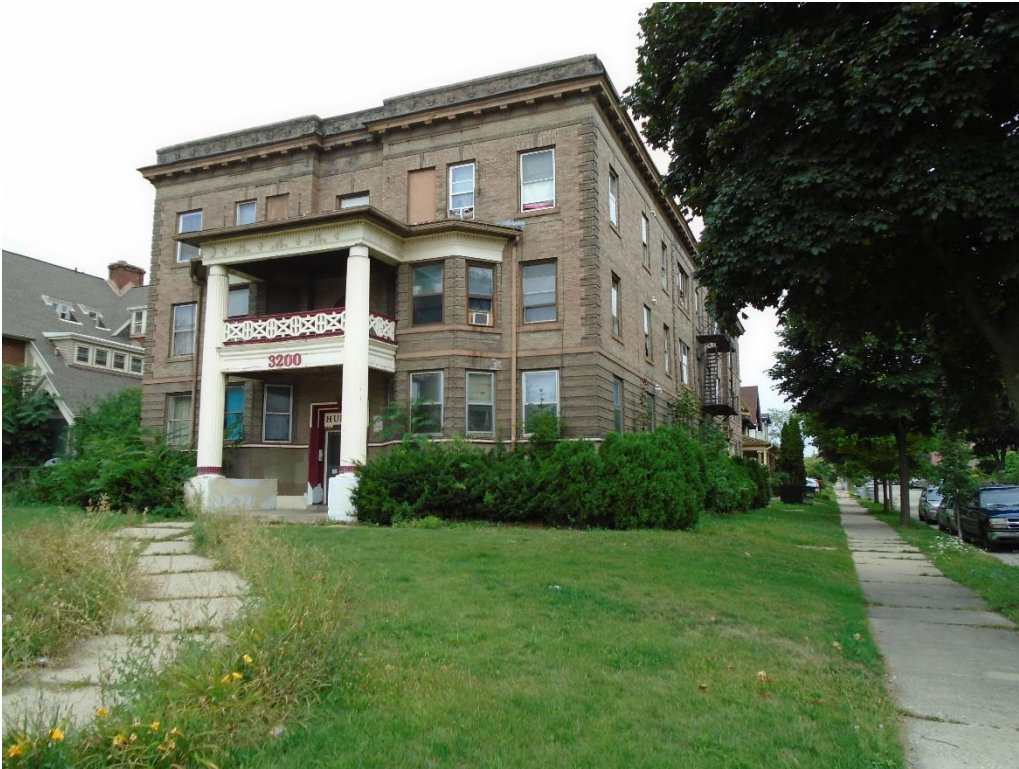
Hudson Flats Apartment Building. Photo taken 2015.
