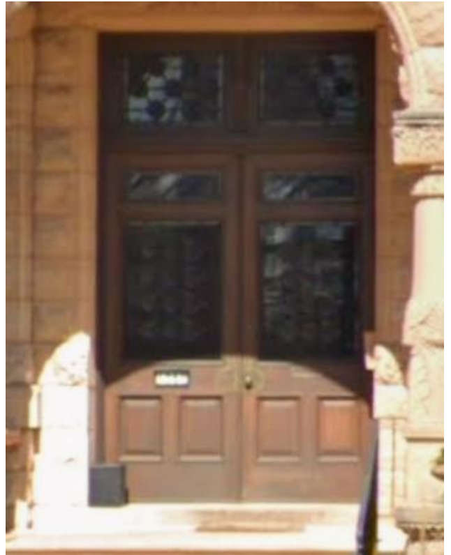
Existing Front Building Entry
