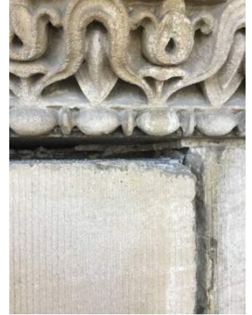
Photo 22 – CARTOUCHE. There are (7) cartouche made up of five elaborately carved stones. Structurally work under compression as the arch over windows, located beneath the solid parapet. North cartouche, upper veneer stone, just above the arch keystone (6" depth). Found condition of displacement, downward action.
