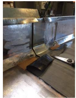
Photo 11 – IN SHOP MOCK-UP. Roofing/flashing tools, ad-hoc expansion joint for review.
