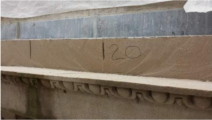
Photo 7 – East elevation. Placement corresponding to field measured stone Dutchman elements.
