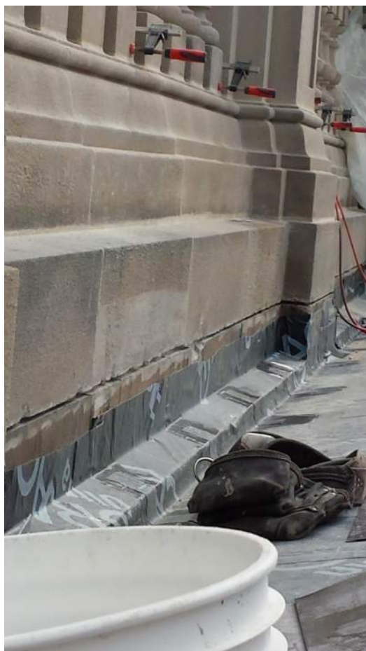
Photo 14 – BALUSTRADE. West elevation at parapet – setting of parapet balusters. Existing balusters replaced the missing and/or damaged balusters at the northwest end elevation. This was for coordination of color, texture in a single bay at the most highly visible elevation.
