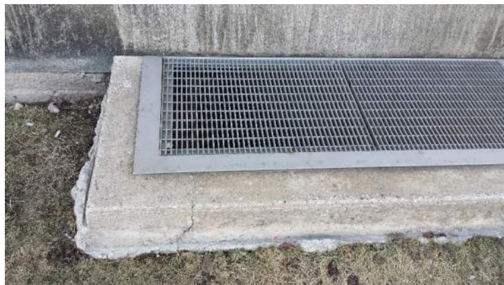
Photo 37 – Window area well grate no. 5, renovated.
