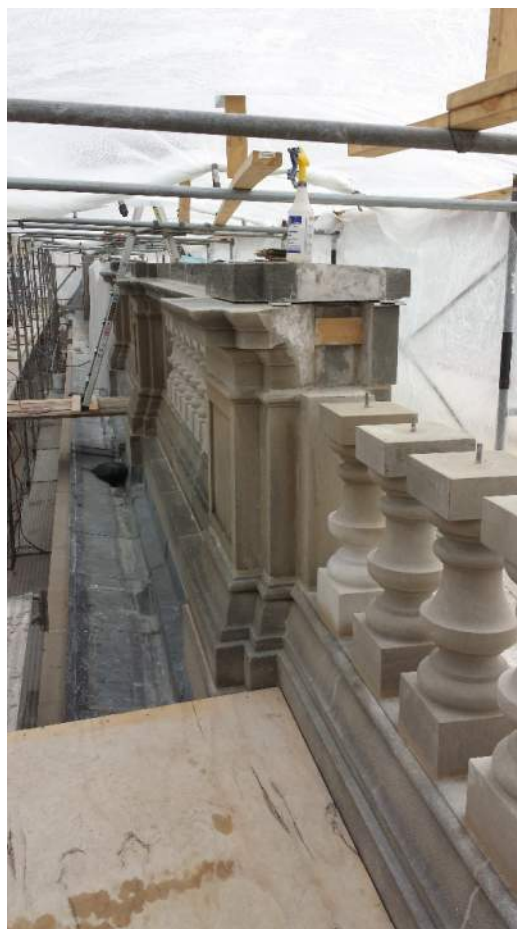
Photo 14 – BALUSTRADE. West elevation at parapet – setting of parapet balusters. Existing balusters replaced the missing and/or damaged balusters at the northwest end elevation. This was for coordination of color, texture in a single bay at the most highly visible elevation.
