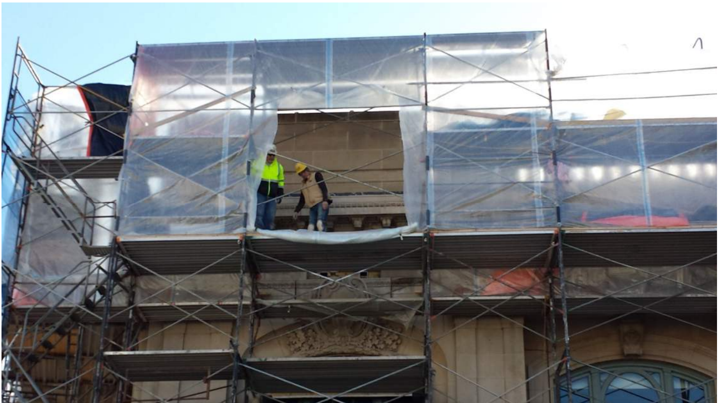
Photo 35 – WEST ELEVATION. Northwest cartouche keystone, repositioned into place.
