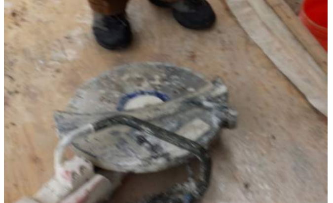
Photo 2 - Hand-sawn, no jig, removal of the damaged cornice gutter edge.
