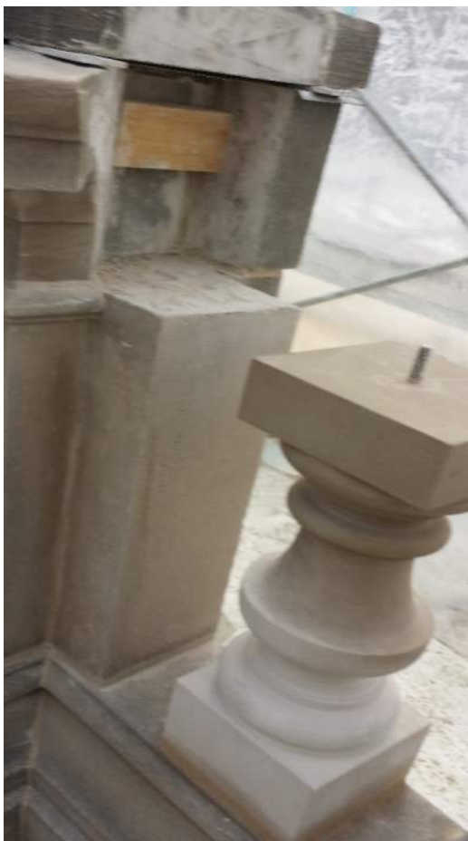
Photo 16 - West elevation. Tradesman tools for cleaning, repointing mortar joints. Severely degraded stones, previously assessed are removed and replaced with carved replicates. Note stainless steel flashing at solid parapet capstone.
