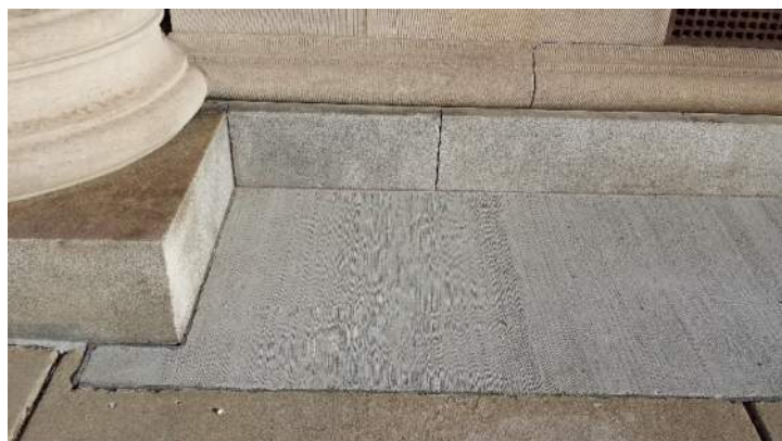
Photo 38 – Window area well grate no. 3 with new concrete cap and concrete support structure beneath. This area well was not draining and in heavy rain conditions would overflow into the lower level storage area. Concrete cap approved by the Historic Preservation Commission and Certificate of Appropriateness released 11/09/2017.
