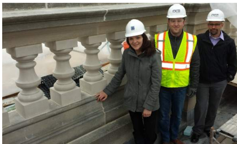
Photo 21 – West elevation, with the new balusters of second bay from the northern end.
