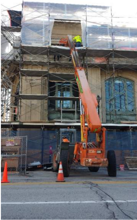
Photos 33, 34 – WEST ELEVATION. Northwest cartouche keystone, repositioned into place with specially fabricated steel hoist system attached to original keystone decoratively carved Indiana limestone block.
