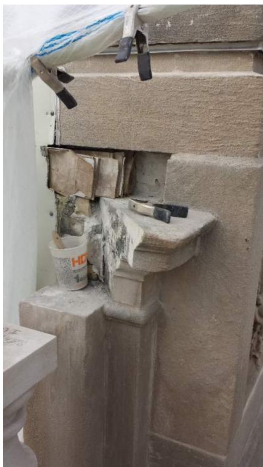
Photo 16 - West elevation. Tradesman tools for cleaning, repointing mortar joints. Severely degraded stones, previously assessed are removed and replaced with carved replicates. Note stainless steel flashing at solid parapet capstone.
