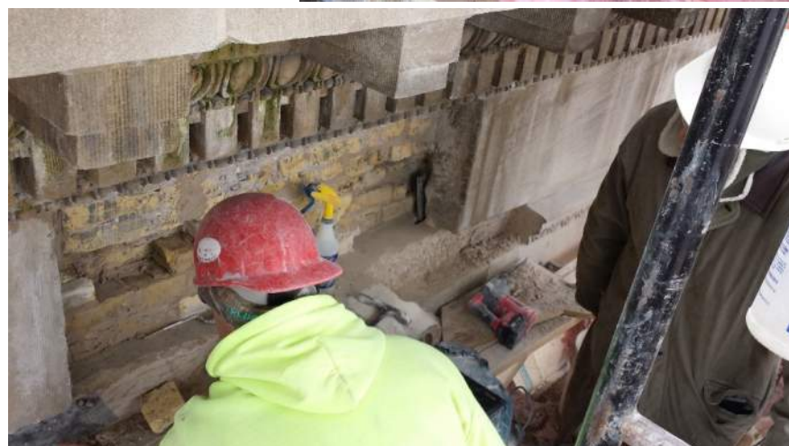
Photo 26 – North cartouche. Brick back-up wall restored, insertion of 0.0375mm steel plates for additional stabilization of facing stone, typical.
