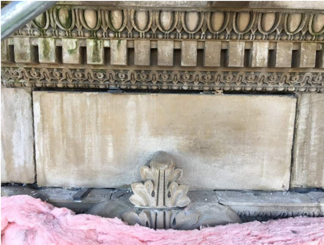
Photo 22 – CARTOUCHE. There are (7) cartouche made up of five elaborately carved stones. Structurally work under compression as the arch over windows, located beneath the solid parapet. North cartouche, upper veneer stone, just above the arch keystone (6" depth). Found condition of displacement, downward action.
