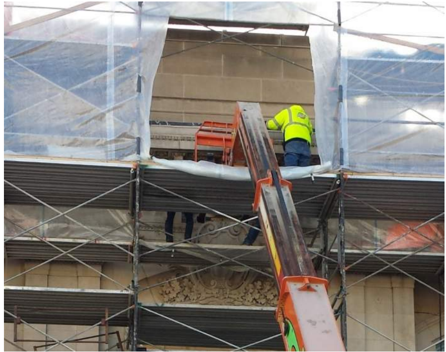
Photos 33, 34 – WEST ELEVATION. Northwest cartouche keystone, repositioned into place with specially fabricated steel hoist system attached to original keystone decoratively carved Indiana limestone block.
