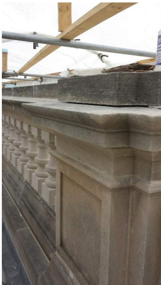
Photo 18 – West elevation. Open parapet railing capstones set. Solid pier cap shimmed for re-setting. Solid pier stones repointed.
