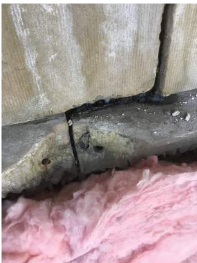
Photo 26 – North cartouche. Brick back-up wall restored, insertion of 0.0375mm steel plates for additional stabilization of facing stone, typical.
