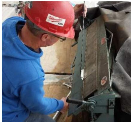
Photo 10 – Roofing/flashing tradesman, bending stainless steel for material development on-site of ad-hoc expansion joint at non-existent cornice drain location.
