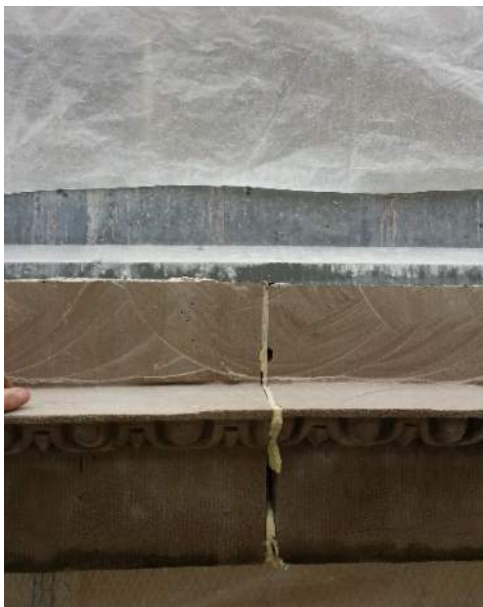
Photo 5 – East elevation. Detail of bare saw-cut and removal.
