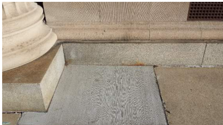
Photo 39 – Window area well no. 2, concrete capped.
