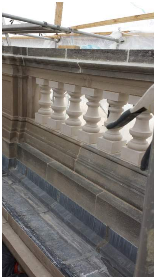
Photo 18 – West elevation. Open parapet railing capstones set. Solid pier cap shimmed for re-setting. Solid pier stones repointed.
