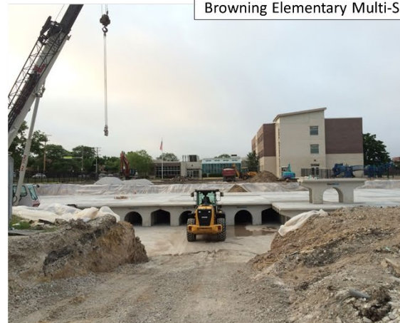
Storm Water Cistern Underneath the Browning Elementary Multi-Sport Court
