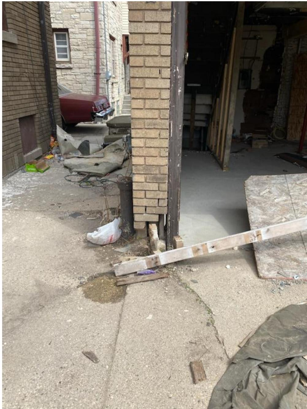
Masonry to be repaired re-using same brick. If additional brick is needed the new brick will match the existing.
