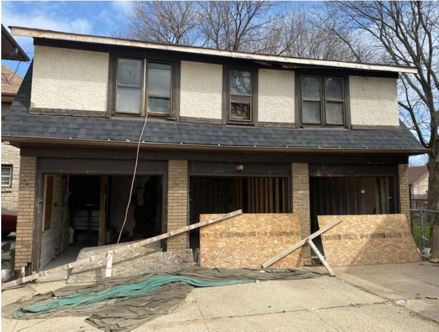
Garage to be repaired including wood trim, wood fascia and wood soffit. At lower left masonry to be repaired.
