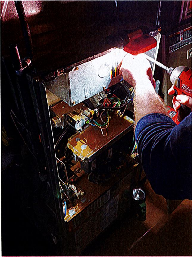
Photo #18: Burkhardt technician examining furnace at 12:00 noon on March 9, 2022).
