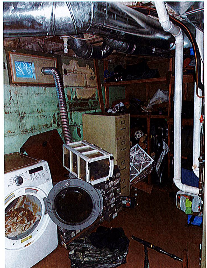
Photo #13: Laundry room; taken at 6:15 a.m. on March 9, 2022).
