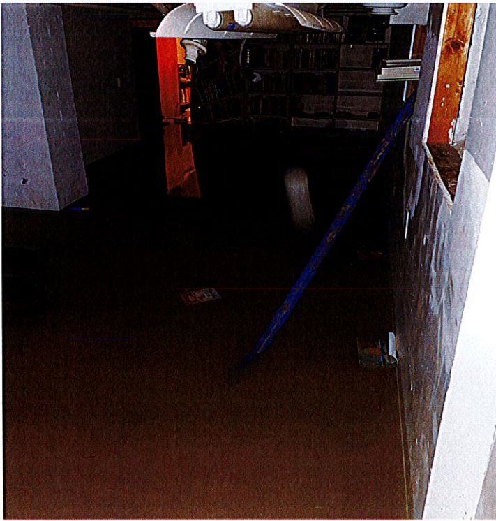
Photo #5: Plumbing company submersible pump continued pumping throughout the night (see blue hose exiting out window). Photo taken at 10:14 p.m. on March 8, 2022.
