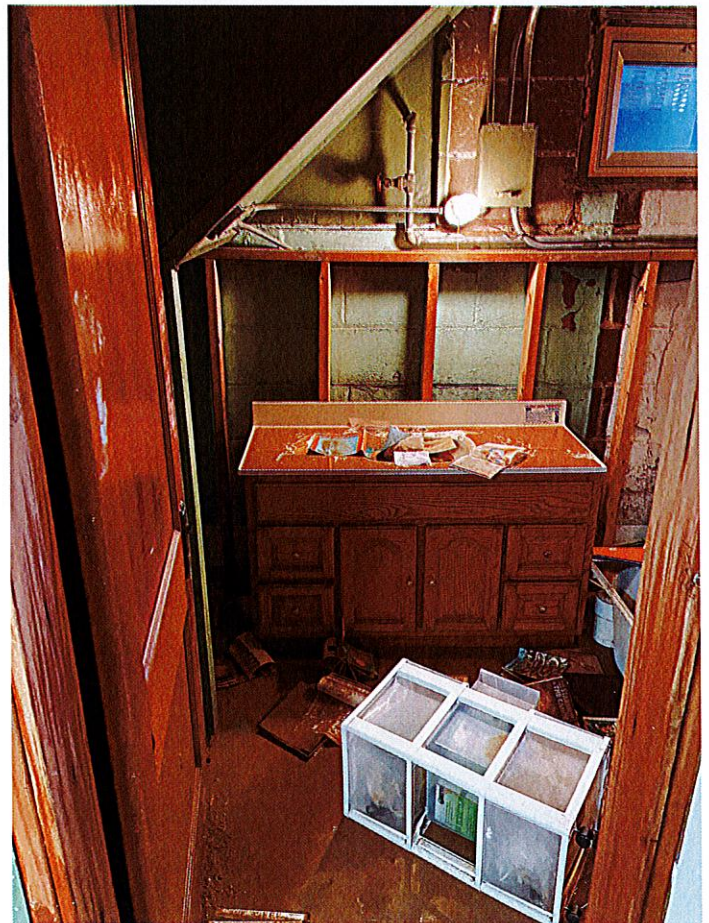
Photo #17: Bathroom; taken at 6:20 a.m. on March 9, 2022).
