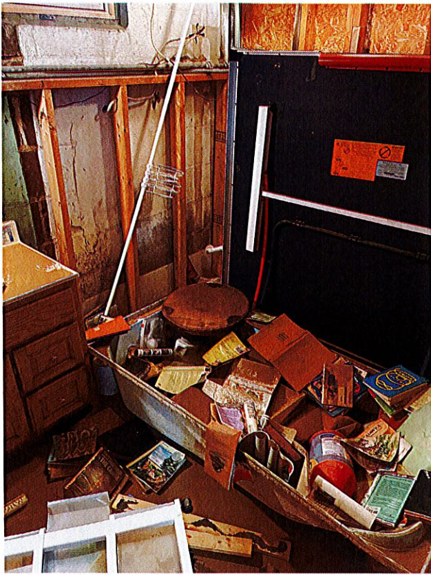
Photo #16: Bathroom; taken at 6:20 a.m. on March 9, 2022).
