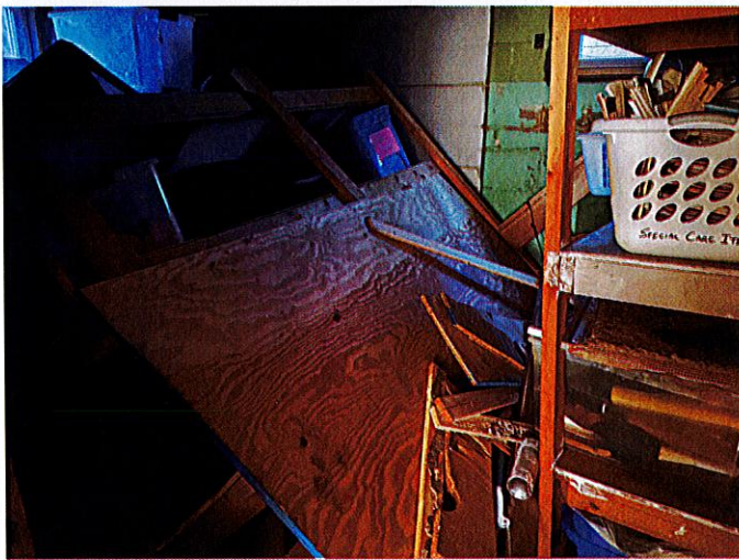
Photo #11: Laundry room; taken at 6:15 a.m. on March 9, 2022).
