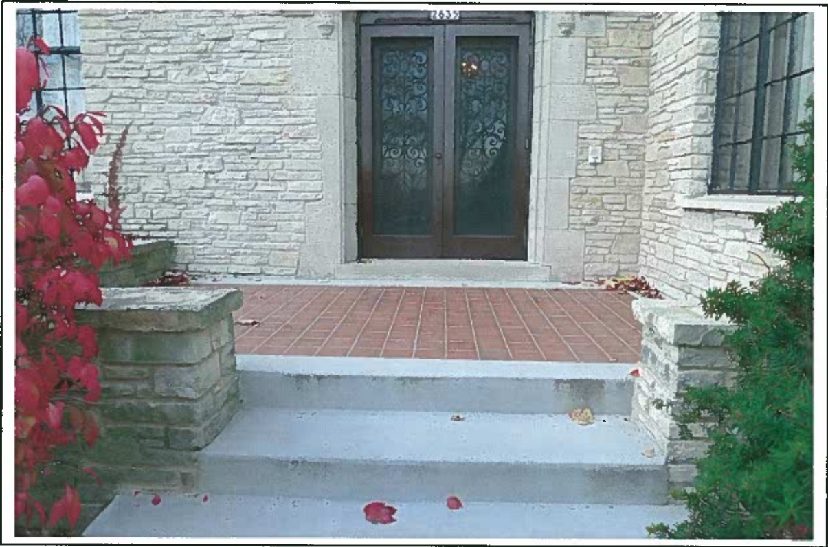
5. Entrance porch with stone wall and tile paving.
