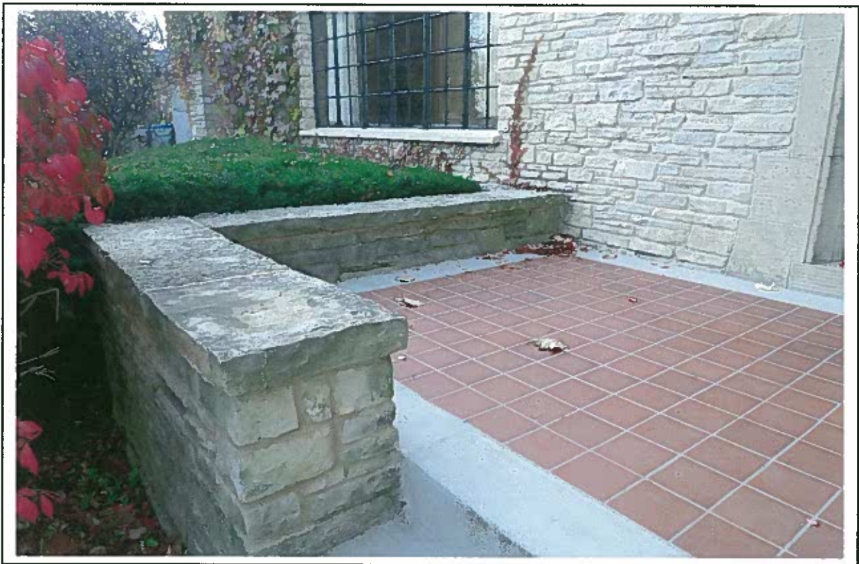
6. South and east section of entrance porch wall.
