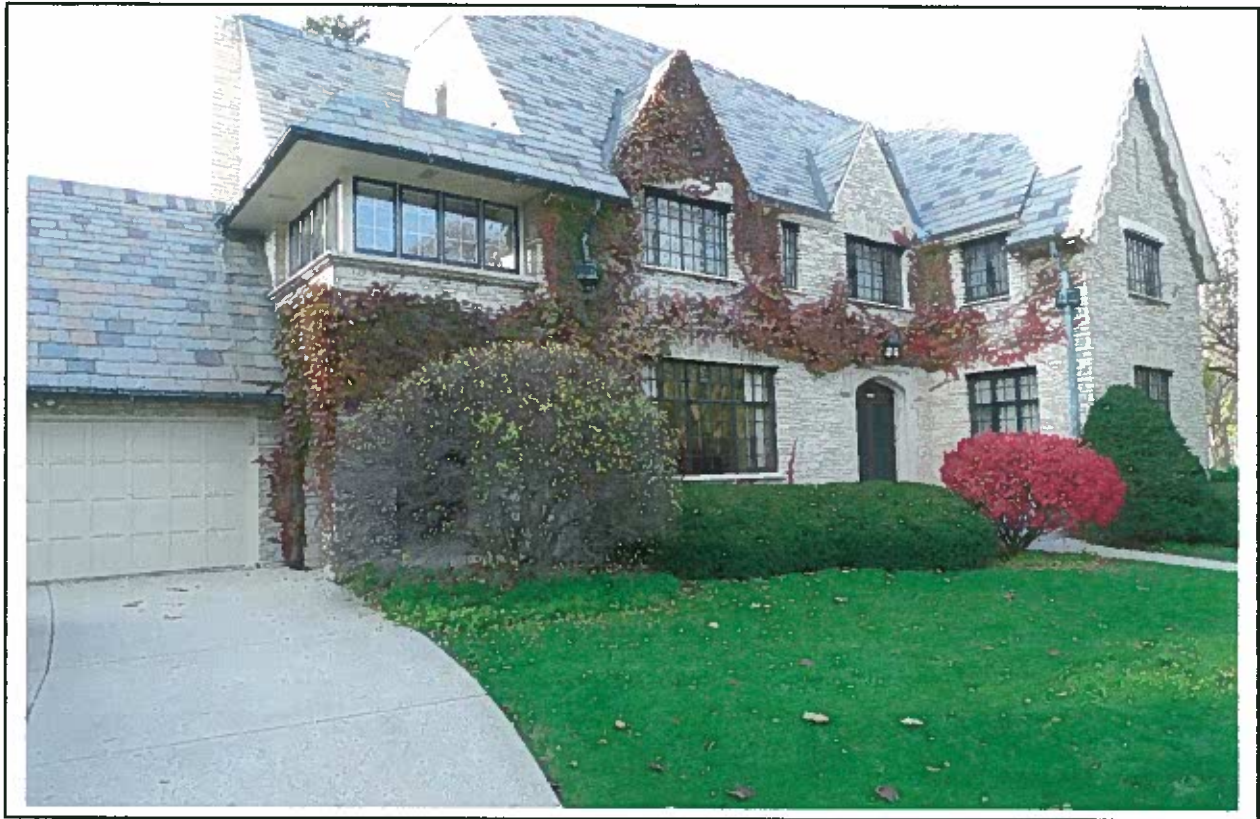
1. Partial view of driveway and southeast corner of house
