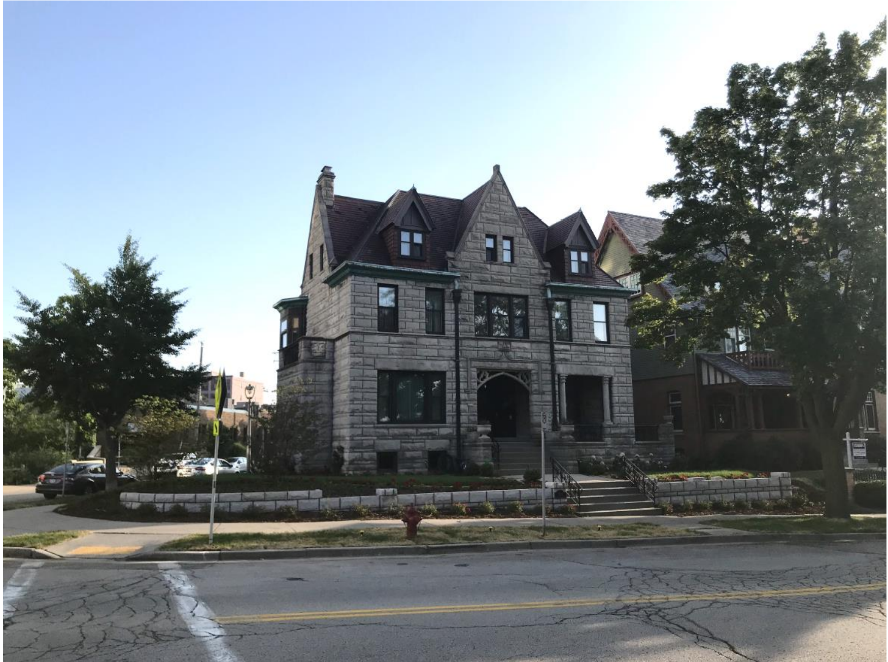
Current condition, masonry columns and masonry seat walls installed
