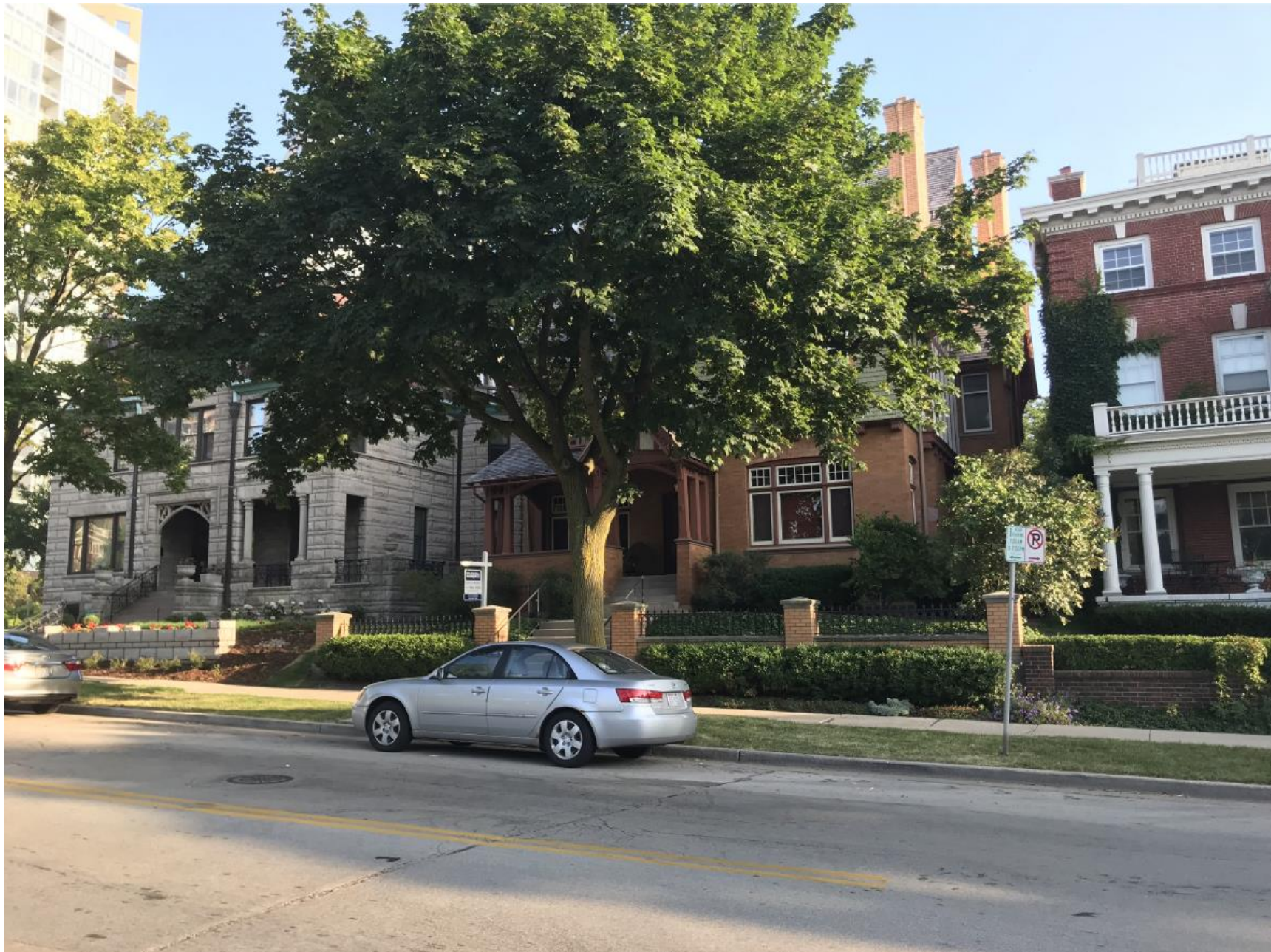
Surrounding context indicating the use of masonry retaining walls along Lafayette
