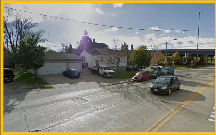
View from West Mineral Street looking south-west (pre-razing)
