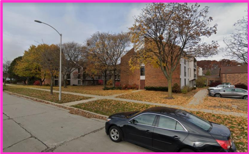
View from W Dean Rd looking north
