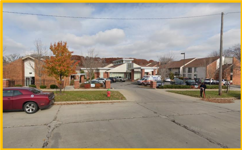
View from W Dean Rd looking north
