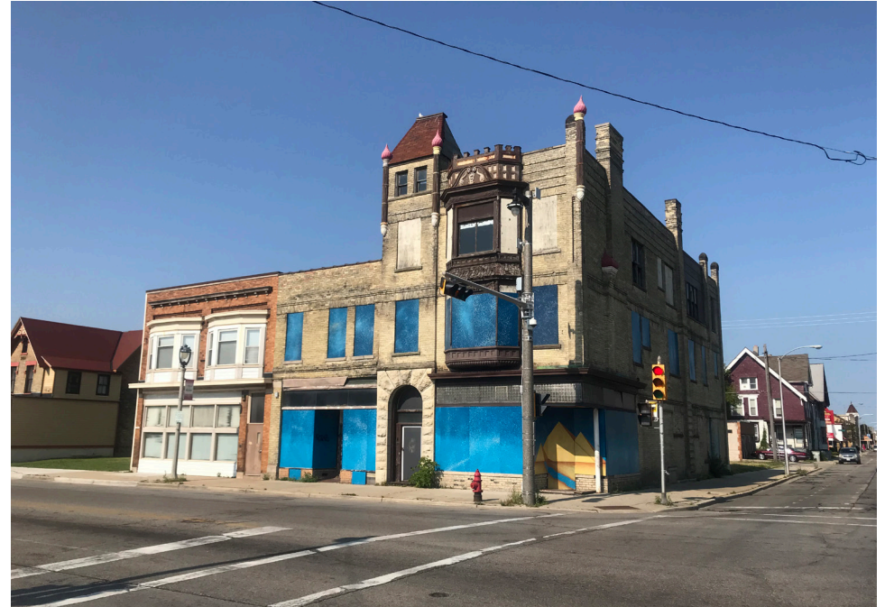
Existing MLK facade
