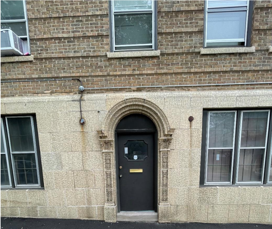
Service entrance on N. 31 st St.
