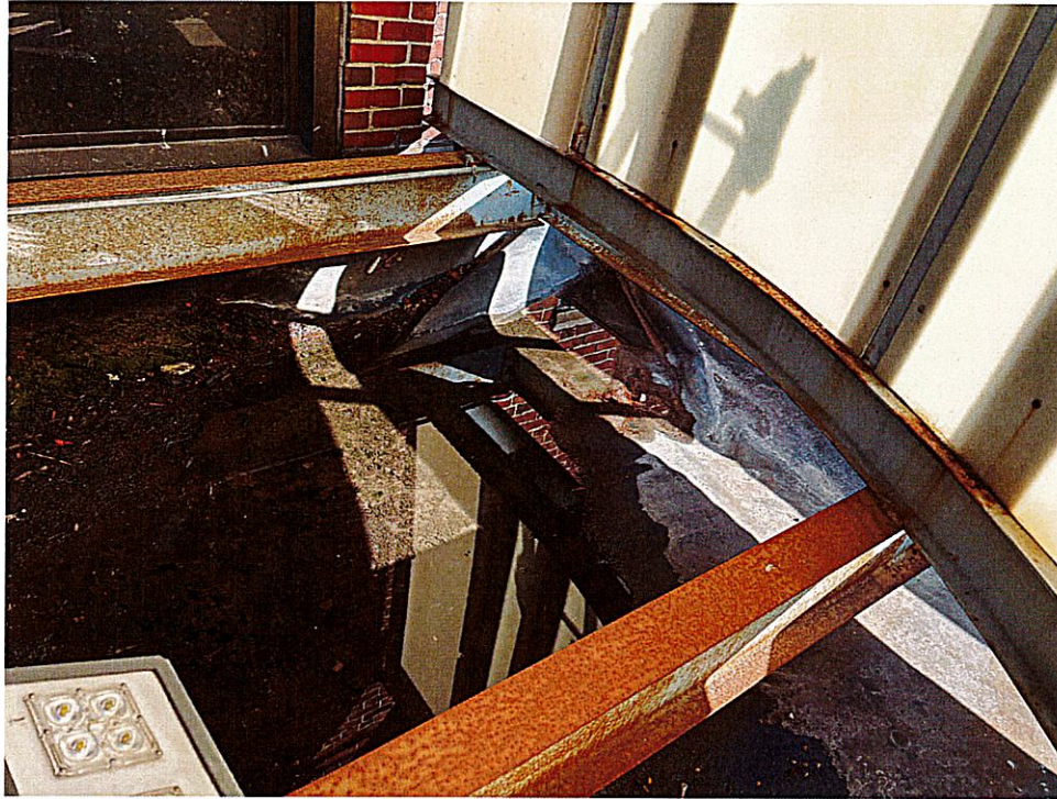
Theatre Roof Section 6 & 8 3.23.26
