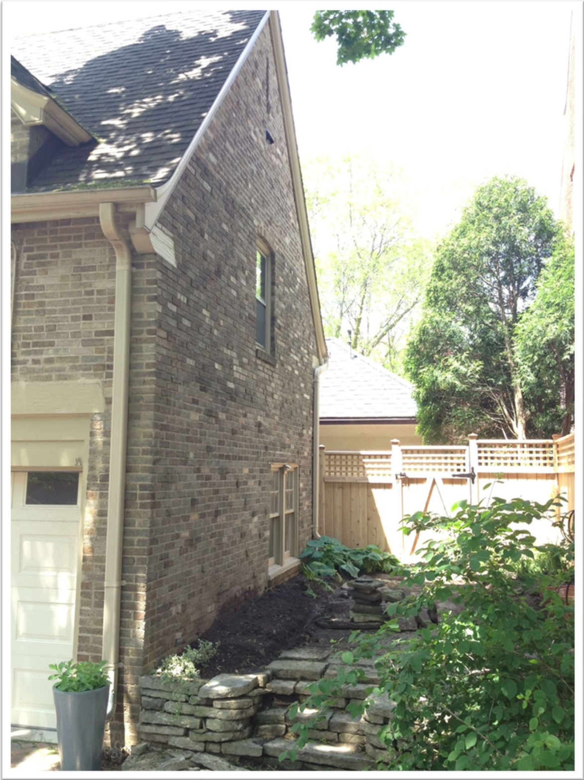
Figure 3. North facade where compressor will be located.
