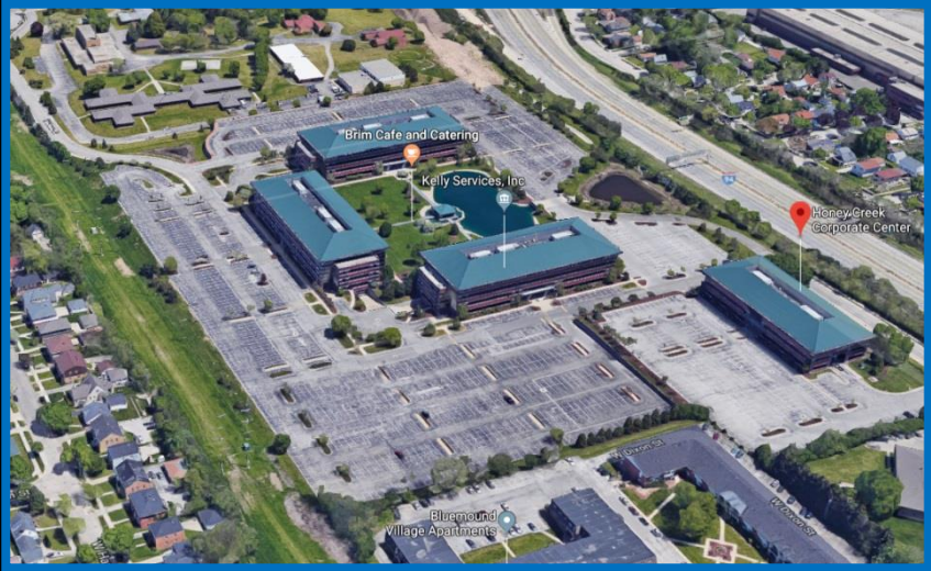
Aerial view looking south-east
