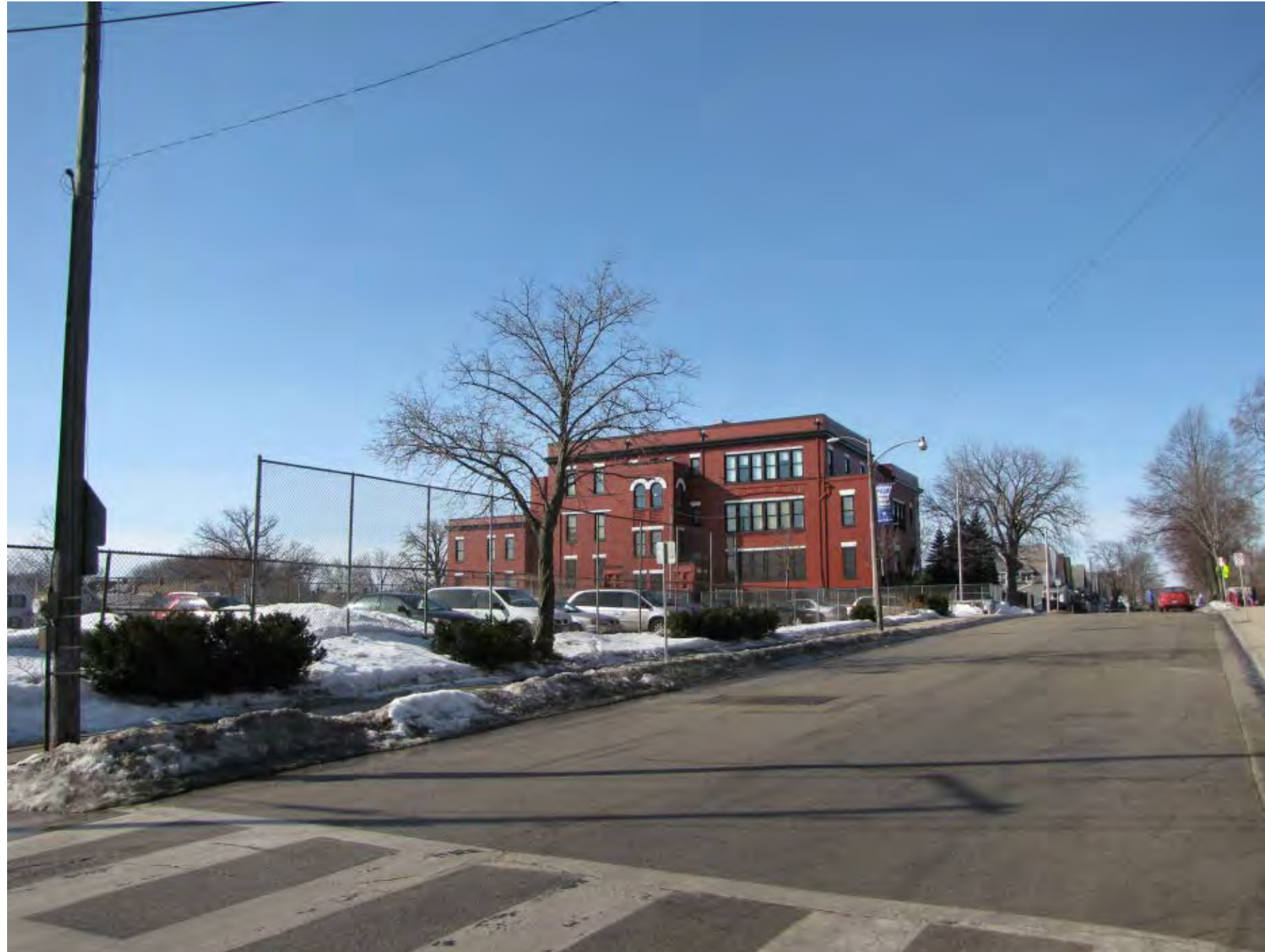
E. DOVER STREET LOOKING WEST AT EXISTING DOVER STREET SCHOOL.
