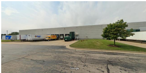
East side of existing building
