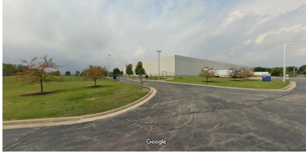
Southeast corner of existing building
