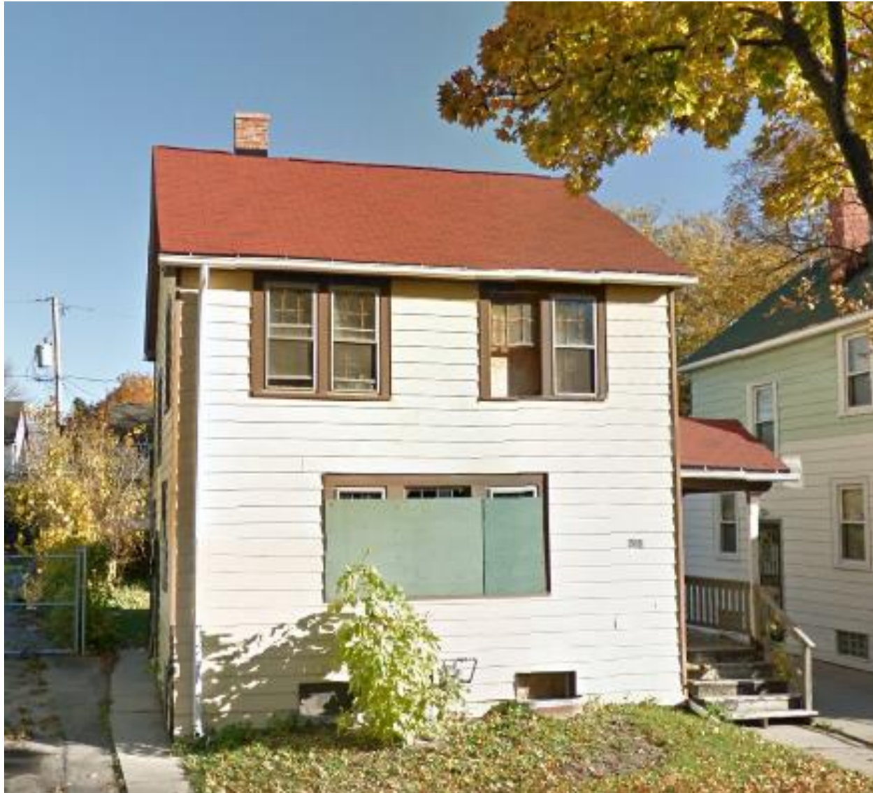
The roof and chimney at 4366 North 26 th street as completed.
