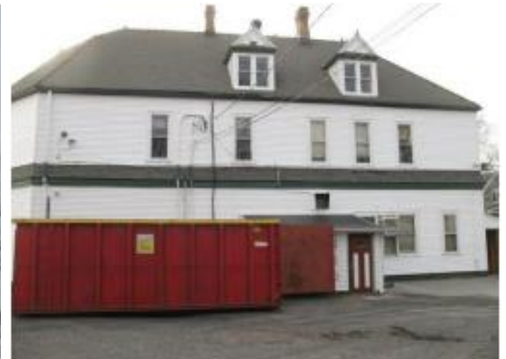
Present condition of rear façade
