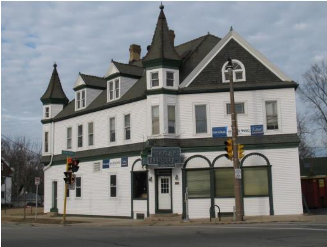
Present condition of front façade
