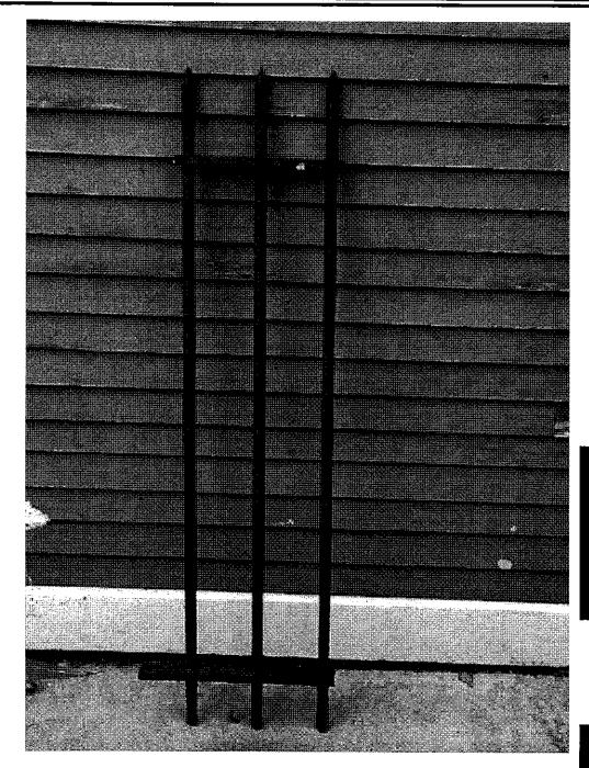
Sample of fence to be installed on south lot line. Sections to be eight feet in length and held in place with square iron posts.
