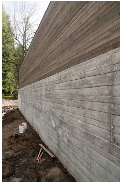
Board Formed Concrete (bottom half) Cedar Wood (top half)
