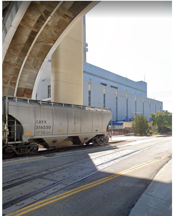
ABOVE RIGHT: WE ENERGIES VALLEY POWER PLANT FACING SOUTHWEST
