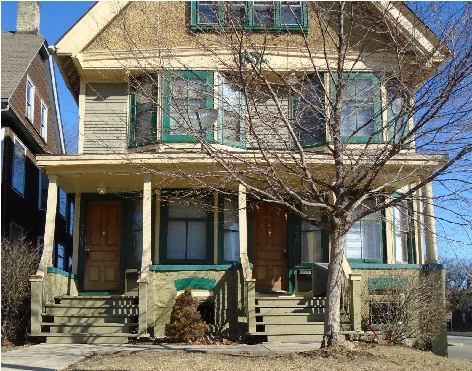
ITEMS 2, 3, 4, & 6. Front Porch, photo of current conditions
