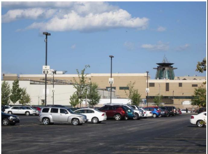
East – Northeast View from Biogas Generation Site
