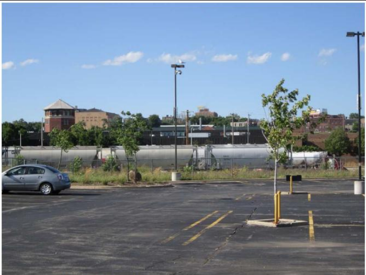
North View from Biogas Generation Site
