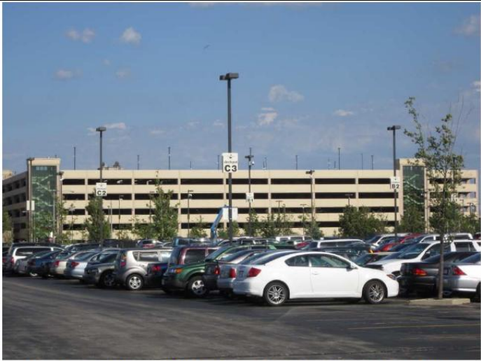
East – Southeast View from Biogas Generation Site
