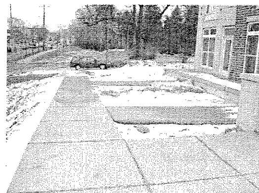
5 RAMP AS-BUILT PICTURE (west view) n.e.
