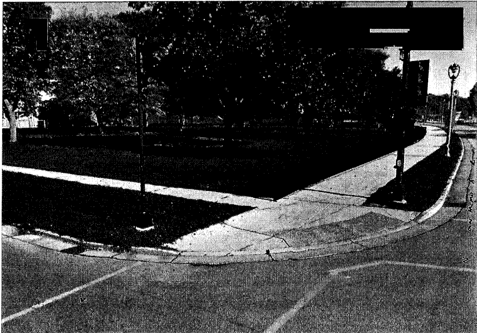
Northwest corner of North Lincoln Memorial Drive and Watertower Road
