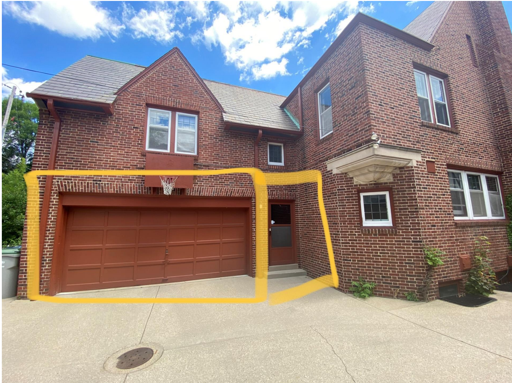
Existing condition. Side door replacement will be reviewed separately.
