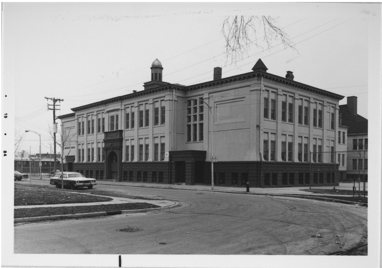
Figure 12: McKinley School, looking southeast, 1984. Source: Wisconsin Architecture and History Inventory.
